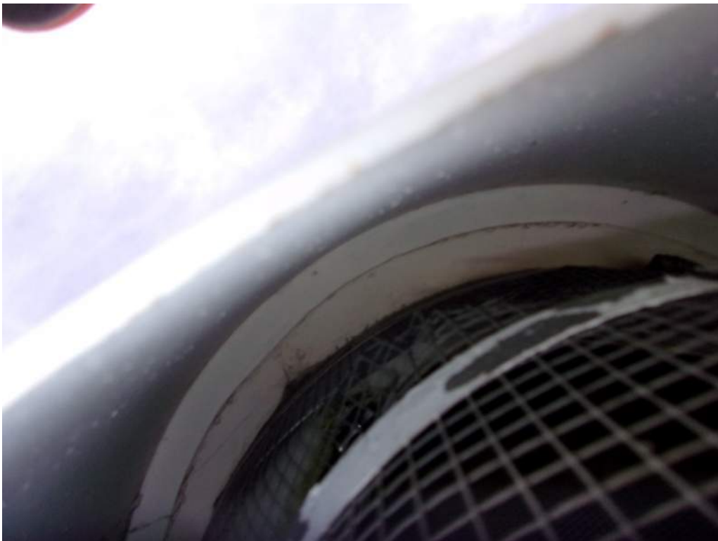
Roof Vent Screen – Not #24
