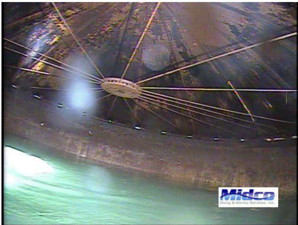
Roof and Support Structure
