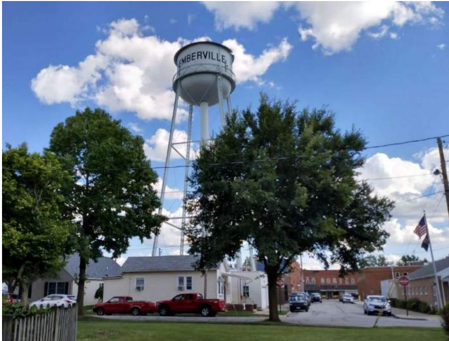
Figure 1 – Pemberville's Existing 100,000 Gallon Water Tower built in 1935
