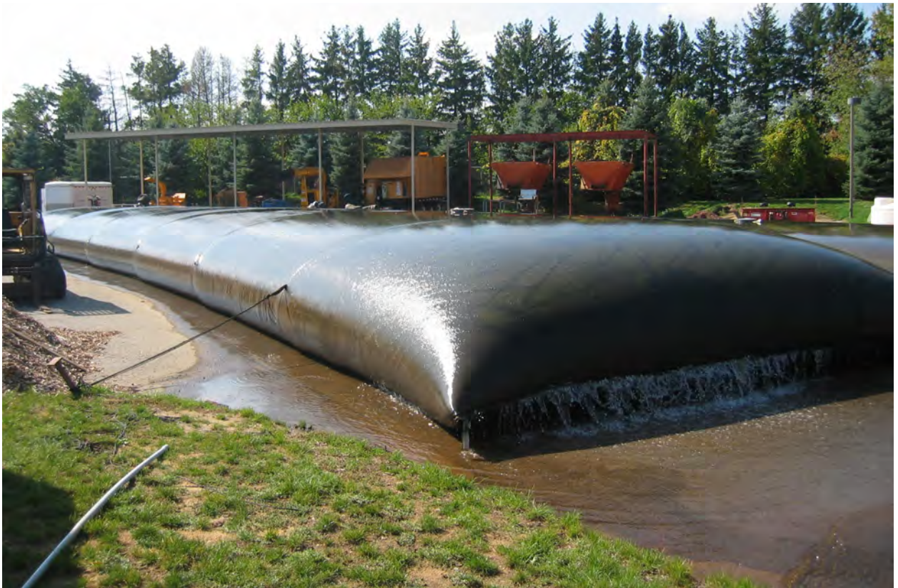
Figure 5. Geotextile bag used for temporary disposal sites with hydraulic dredging.
