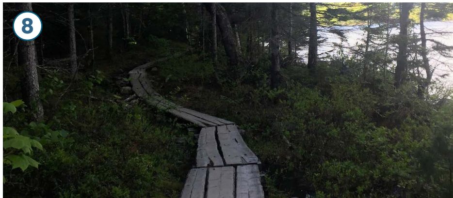
Example boardwalk through wetlands
