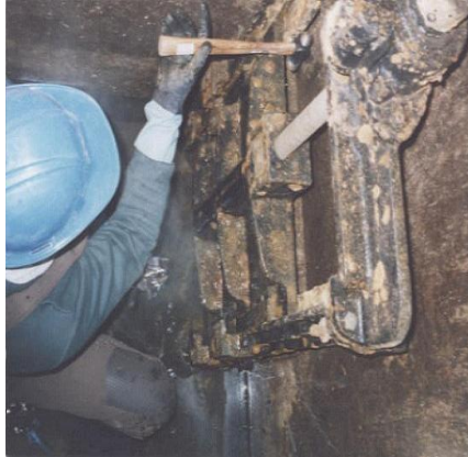
Slide Gate Repair Bad Axe 33
