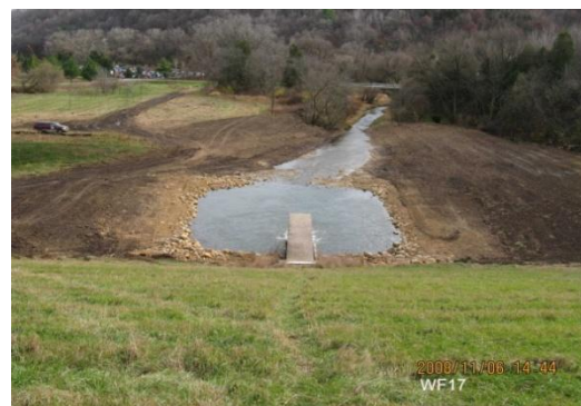
West Fork 17 Stilling Basin Repair – Oct. 2008
