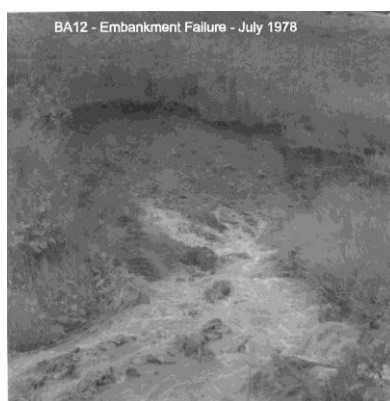
Near-Failure of Bad Axe 12 (Runge Hollow) 1978
