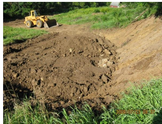
West Fork 12 Aux. Spwy Repair – July 2008
