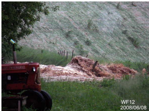
West Fork 12 Overtopping – June 2008
