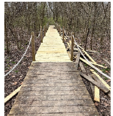
Right: Interior trail bridge repairs.
