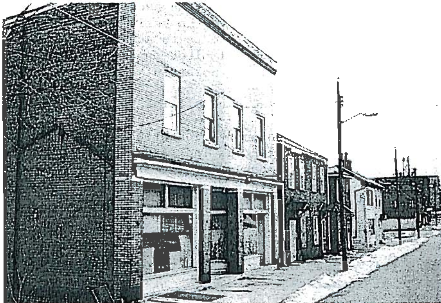
The foreground building, a well-preserved example of a neighborhood-scale commercial structure, is in the traditionally Polish neighborhood above (west of) North Seventh Street near North and Highland.
