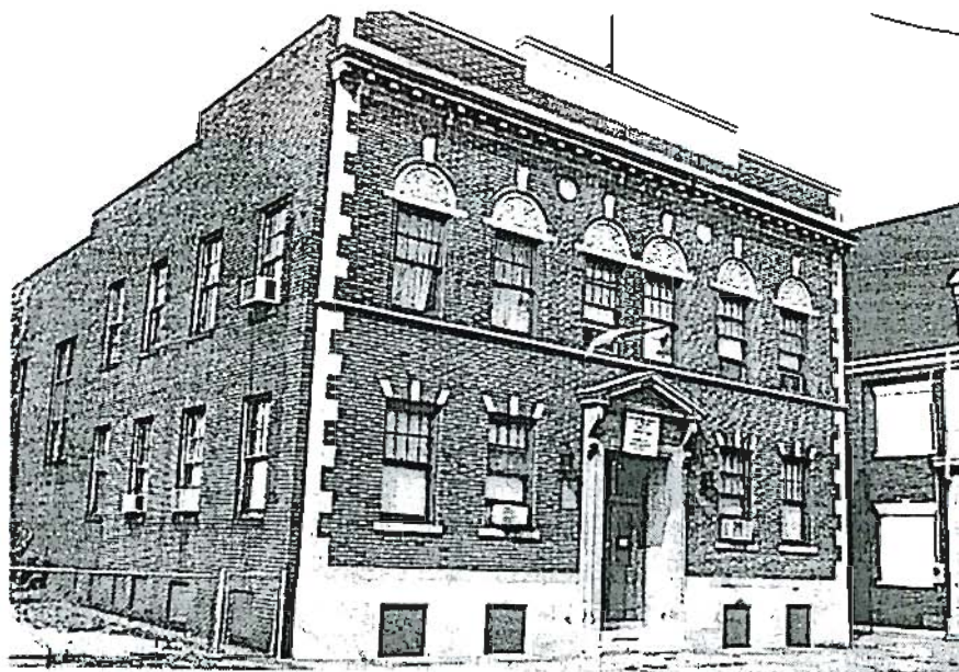
The Jefferson County War Memorial Building on North Street is another good example of civic architecture. Both it and the Post Office exhibit classical detailing.
