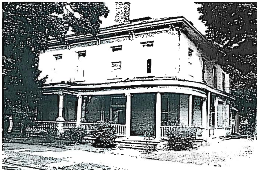
A late-nineteenth century double at 328-332 South Fourth Street has Italianate detailing and a handsome early twentieth century Colonial Revival porch.
