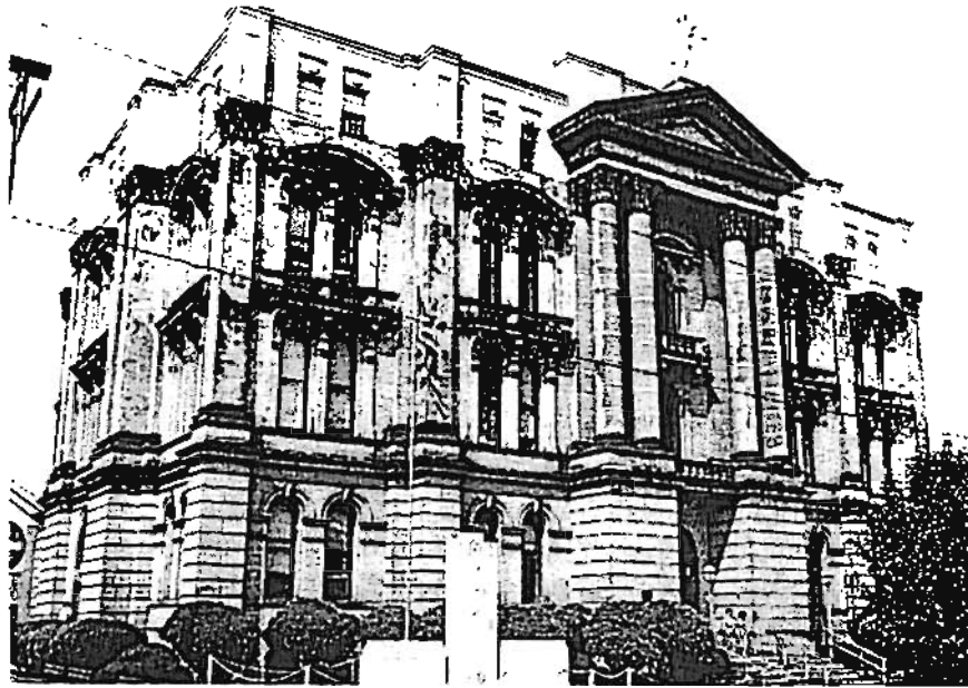
The Jefferson County Courthouse, though much altered, still has a commanding presence at the corner of Third and Market Streets.
