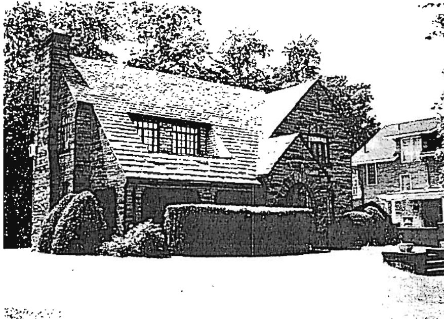
The early 20th century stone house at 309 Lawson Avenue in Pleasant Heights exemplifies the attention to style, appearance, and details that was important to owners of the more expensive subdivision houses.
