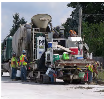
McLean Boulevard reconstruction nears completion.
