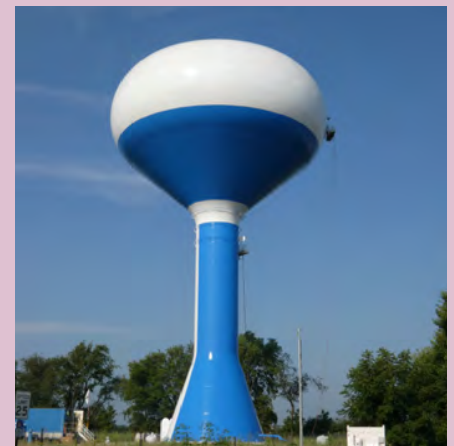
The new water tower at Kingsport and Lone Drive will store 1.25 million gallons.
