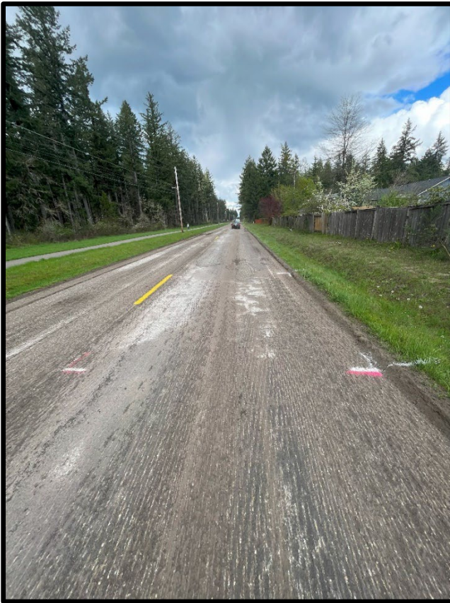
5-8-2023: Roadway leveling/milling complete.
