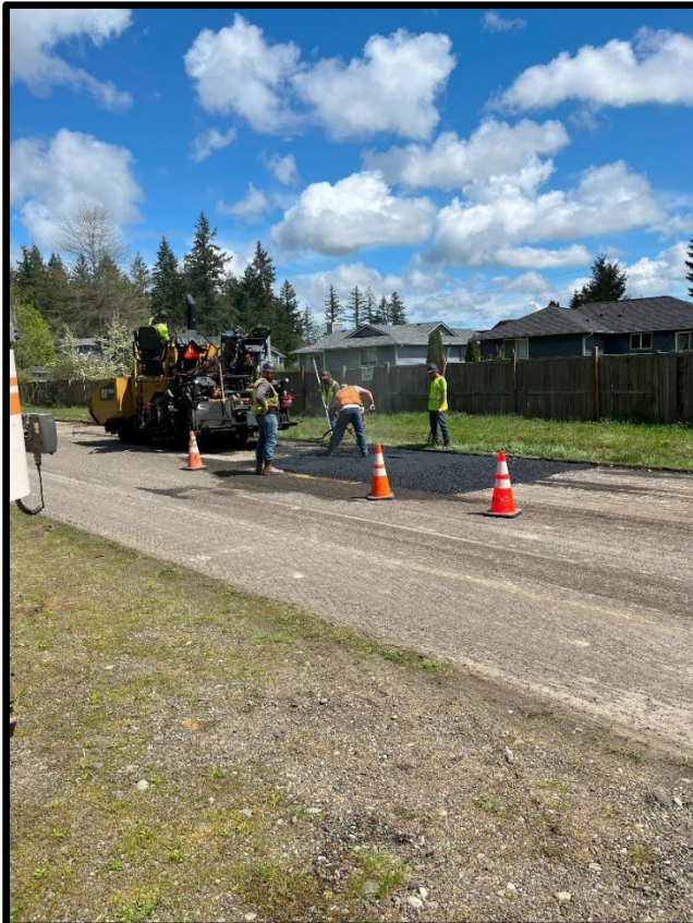
5-9-2023: Pavement Removal and Soft Spot Repair
