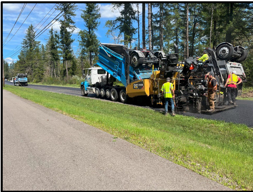
5-10-2023: Paving the 2" Asphalt Concrete Overlay
