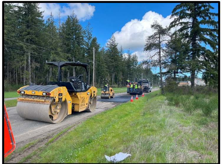
5-9-2023: Pavement Removal and Soft Spot Repair
