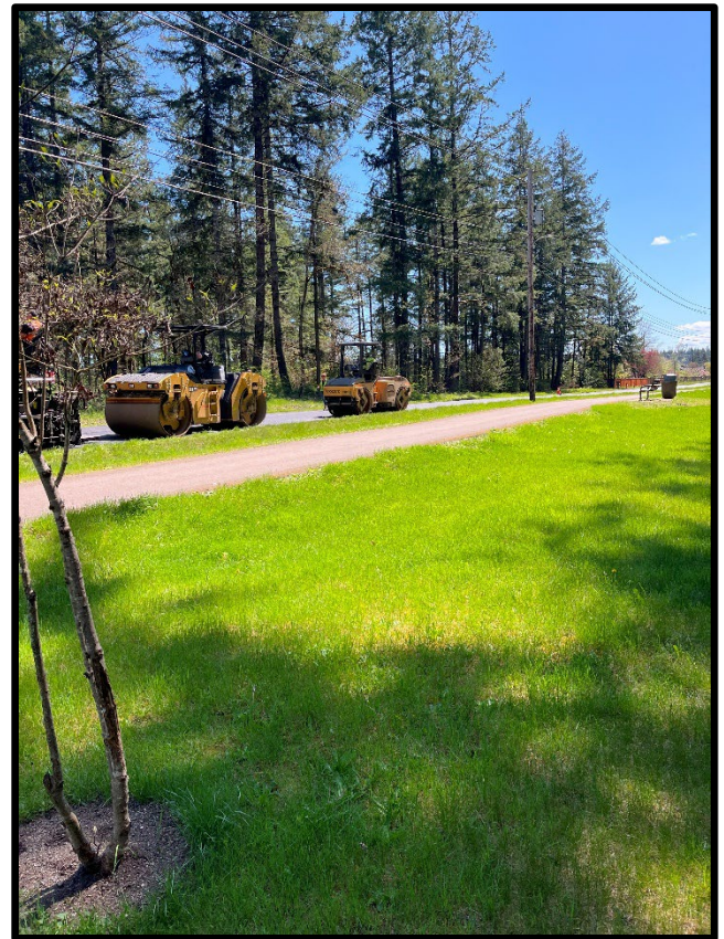
5-10-2023: Compaction of A.C. Overlay
