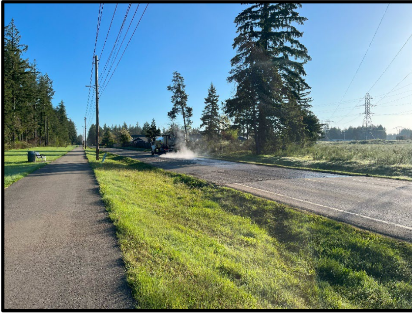
5-10-2023: Asphalt Emulsion Tack Coat Application
