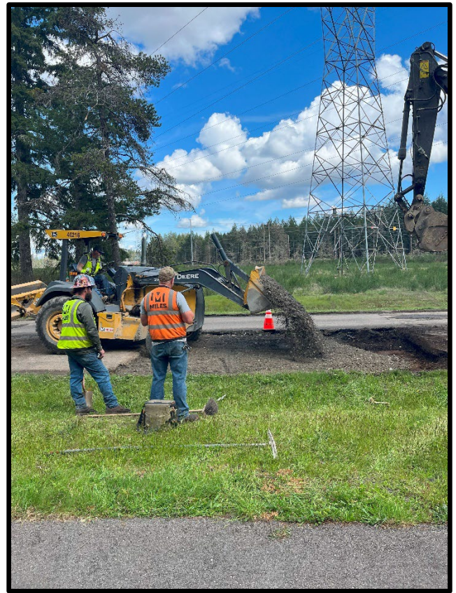
5-9-2023: Pavement Removal and Soft Spot Repair
