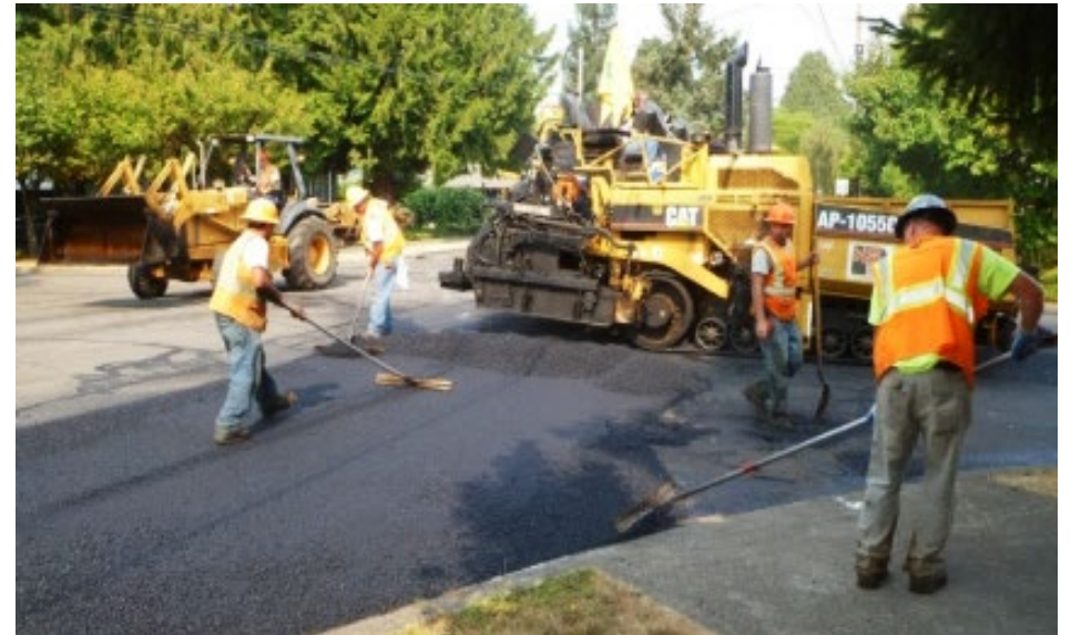
2021 Park Street pavement overlay
