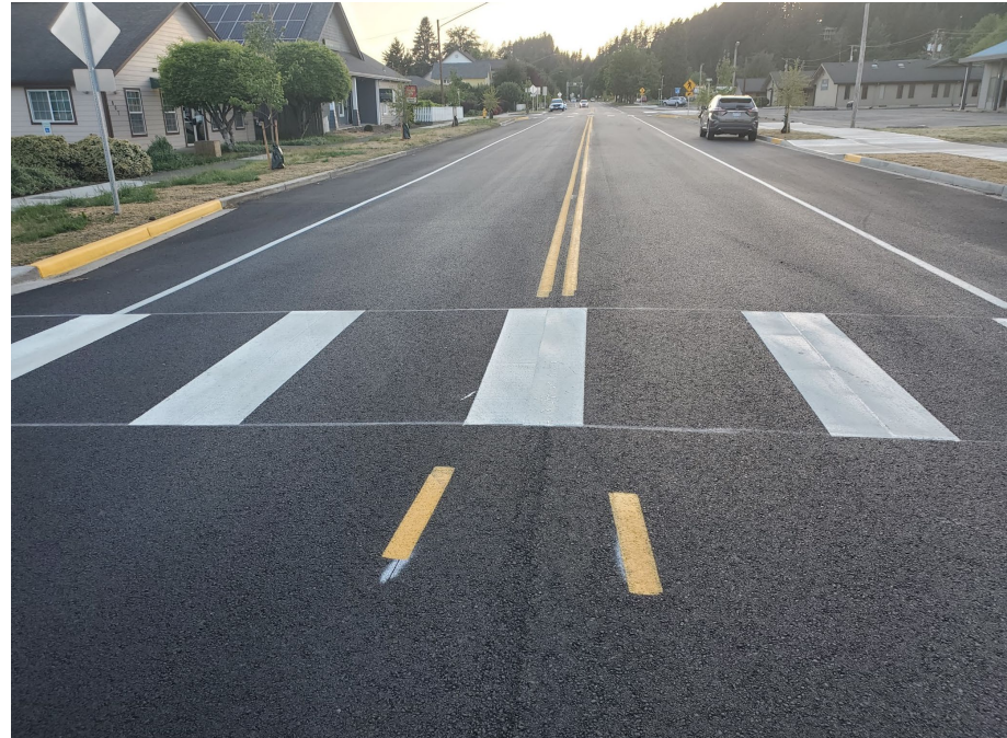
Western Gateway – Railroad Avenue Paving and Pedestrian Improvements
