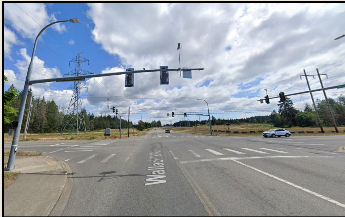
Signal at Wallace Kneeland Blvd. & Shelton Springs Road.
