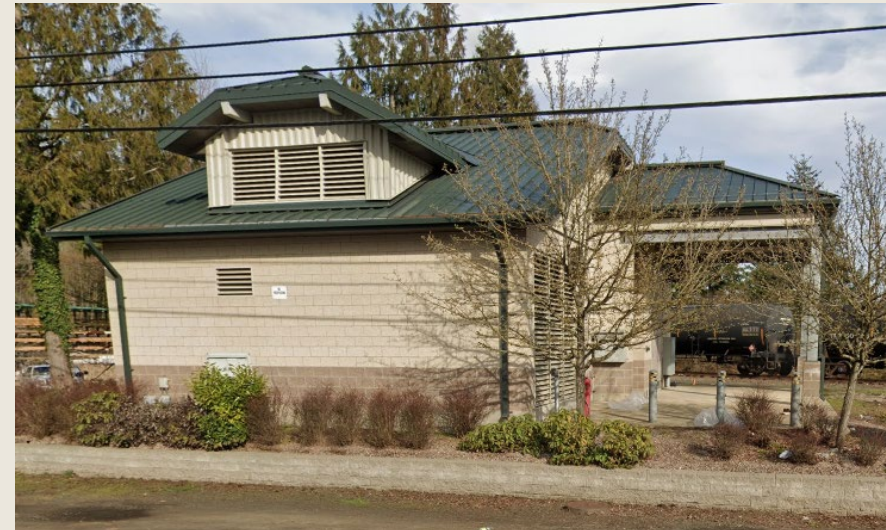
Front Street Lift Station
