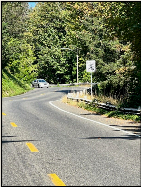
Highland Drive Guardrail
