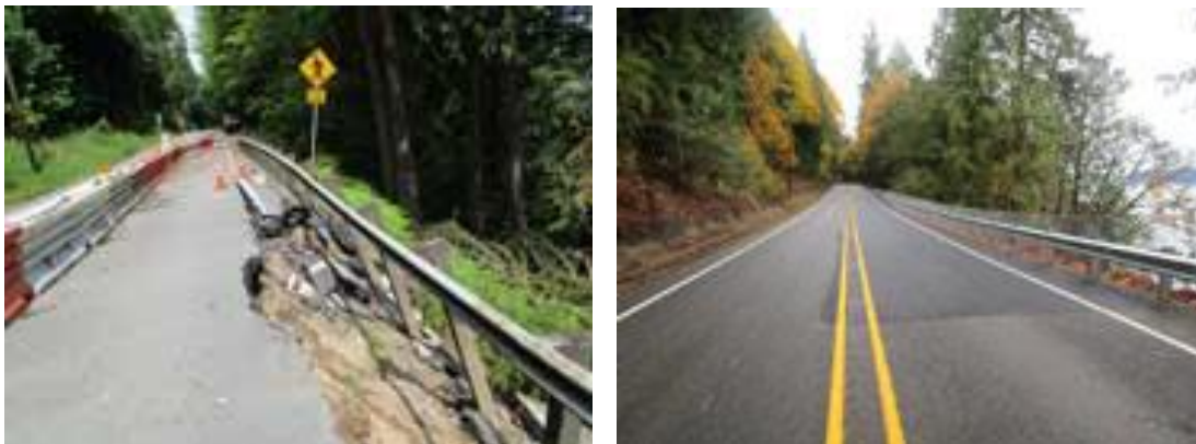
Figure 8-10 Before and After Pictures of SR 101/ 2.2 miles South of Beacon Pt. Road
