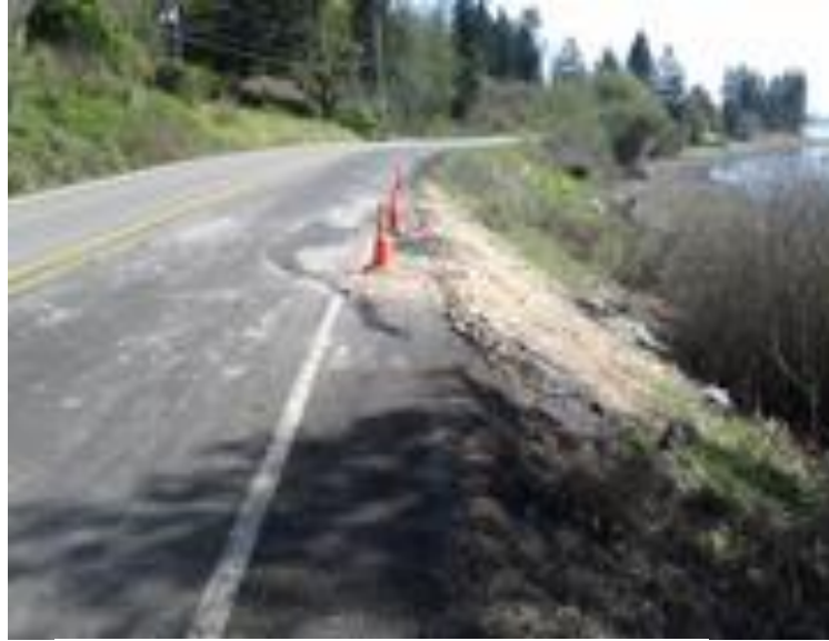
Figure 8-11 SR 302 Slope Erosion Near Victor
