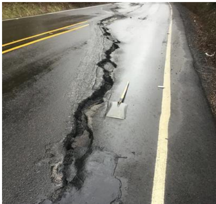
Figure 8-12 Highway 302 Landslide East of Victor (2022)
