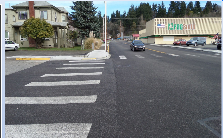
1 st Street Improvements
