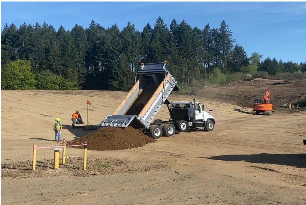
Photograph 6. Construction of foundation layer on Property. Wells AMW-02 and AMW-03 are shown. Photo faces west-northwest.
