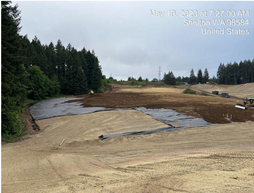
Photograph 7. Installation of geotextile barrier. Photo faces north-northeast.
