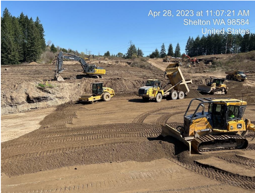
Photograph 5. Backfill and compaction of landfill waste relocation excavation on south-adjacent property. Photo faces north.
