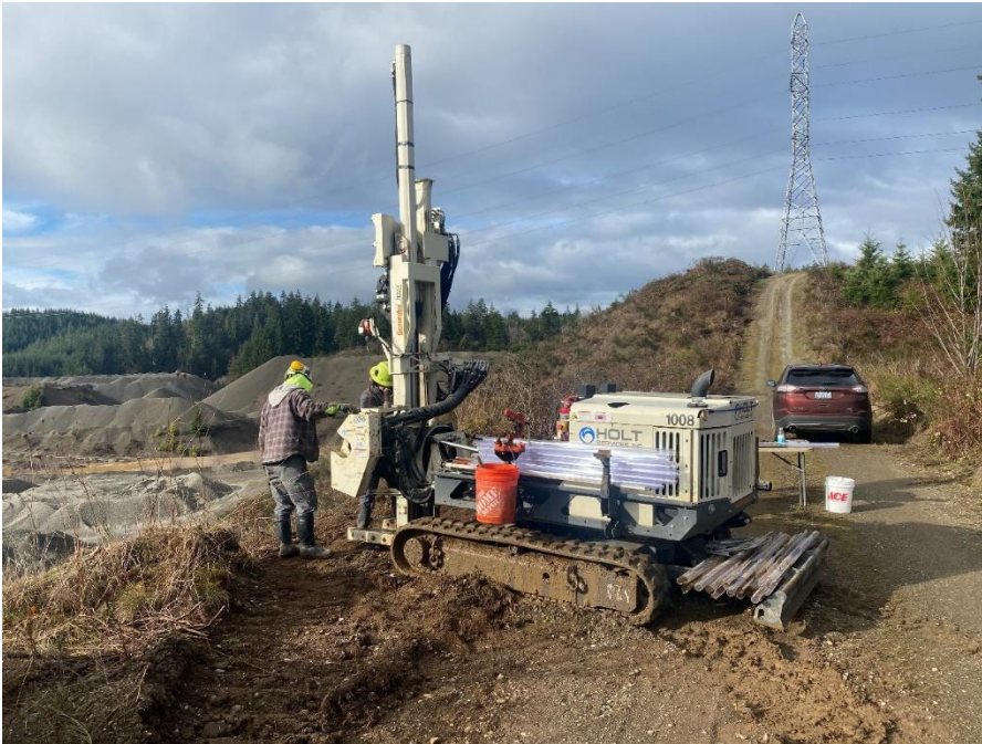
Photograph 3. Exploratory drilling on the south-adjoining property to delineate the extent of landfill waste beyond the south Property boundary. Photo faces west.
