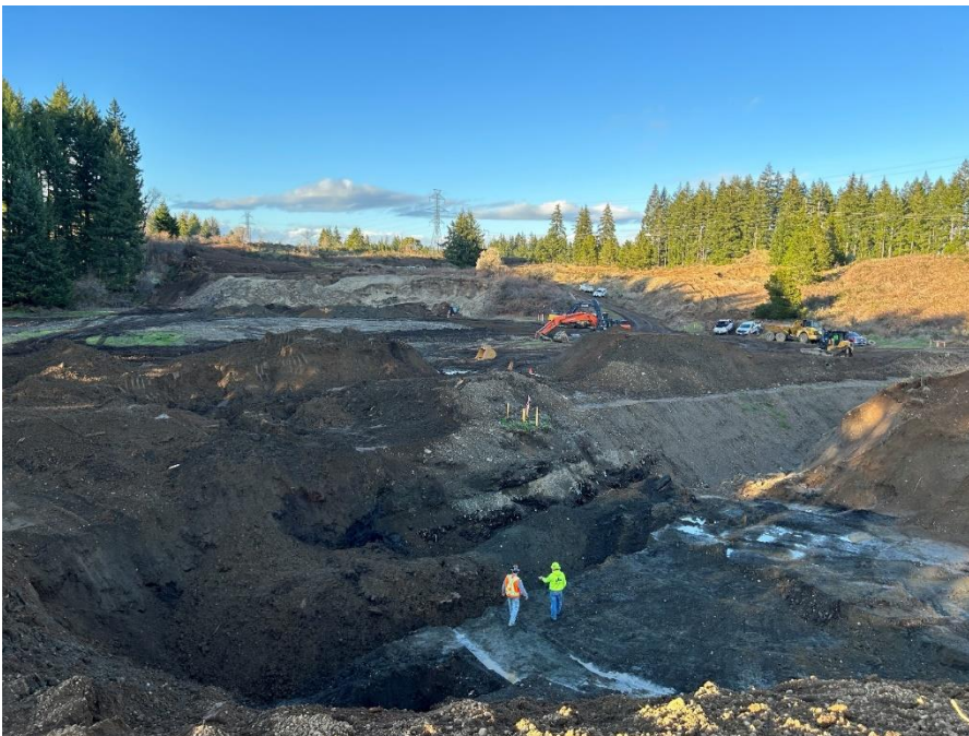
Photograph 4. Landfill waste relocation excavation on south-adjoining property. Landfill waste shown in dark-colored layers. Photo faces north.
