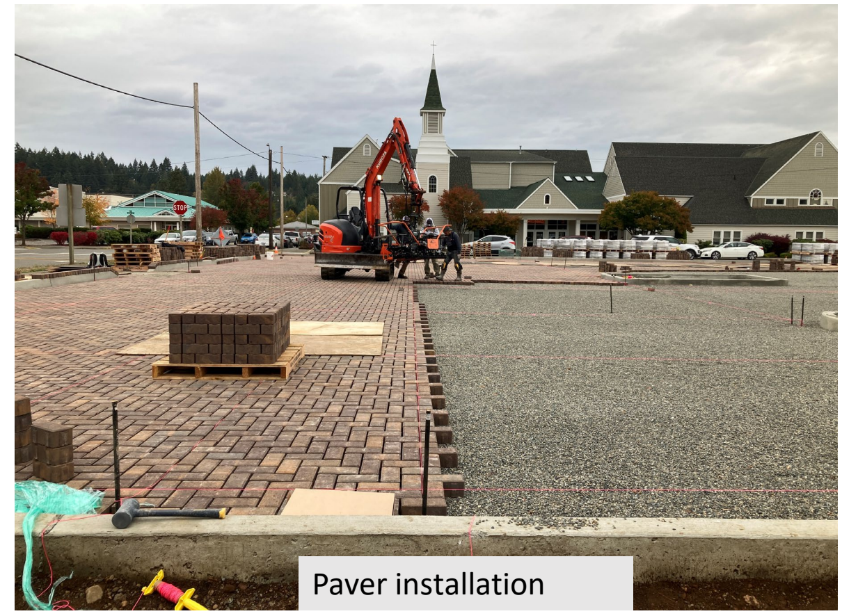
Start of paver installation
