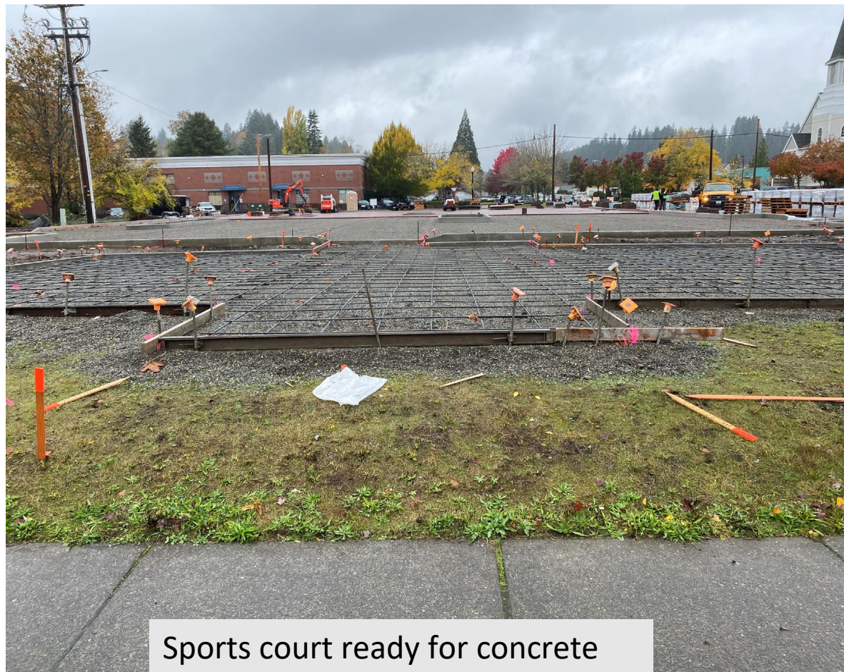
Pouring concrete flatwork
