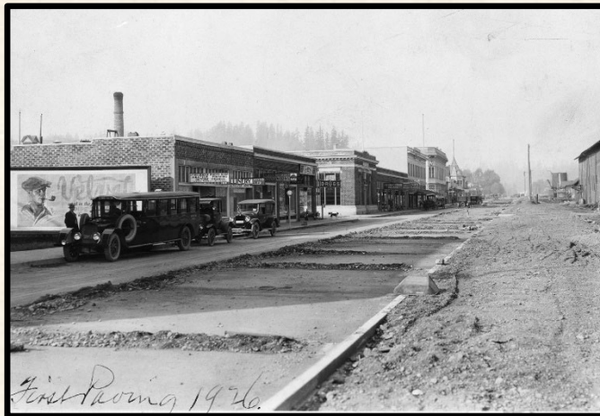
1926 First Roadway Paving
