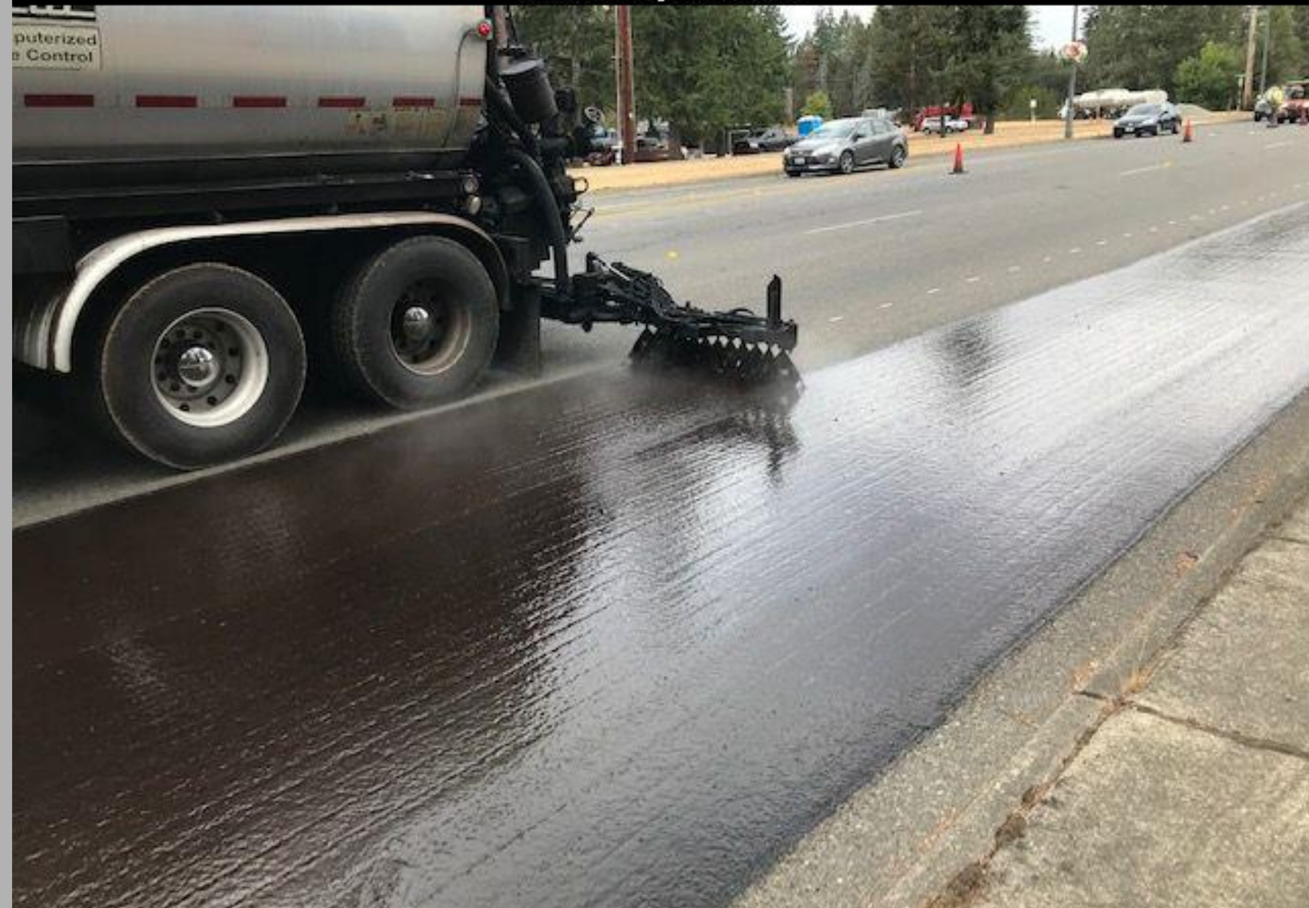
Placing emulsified asphalt in bus stop on N13th in front of Olympic College prior to rock placement
