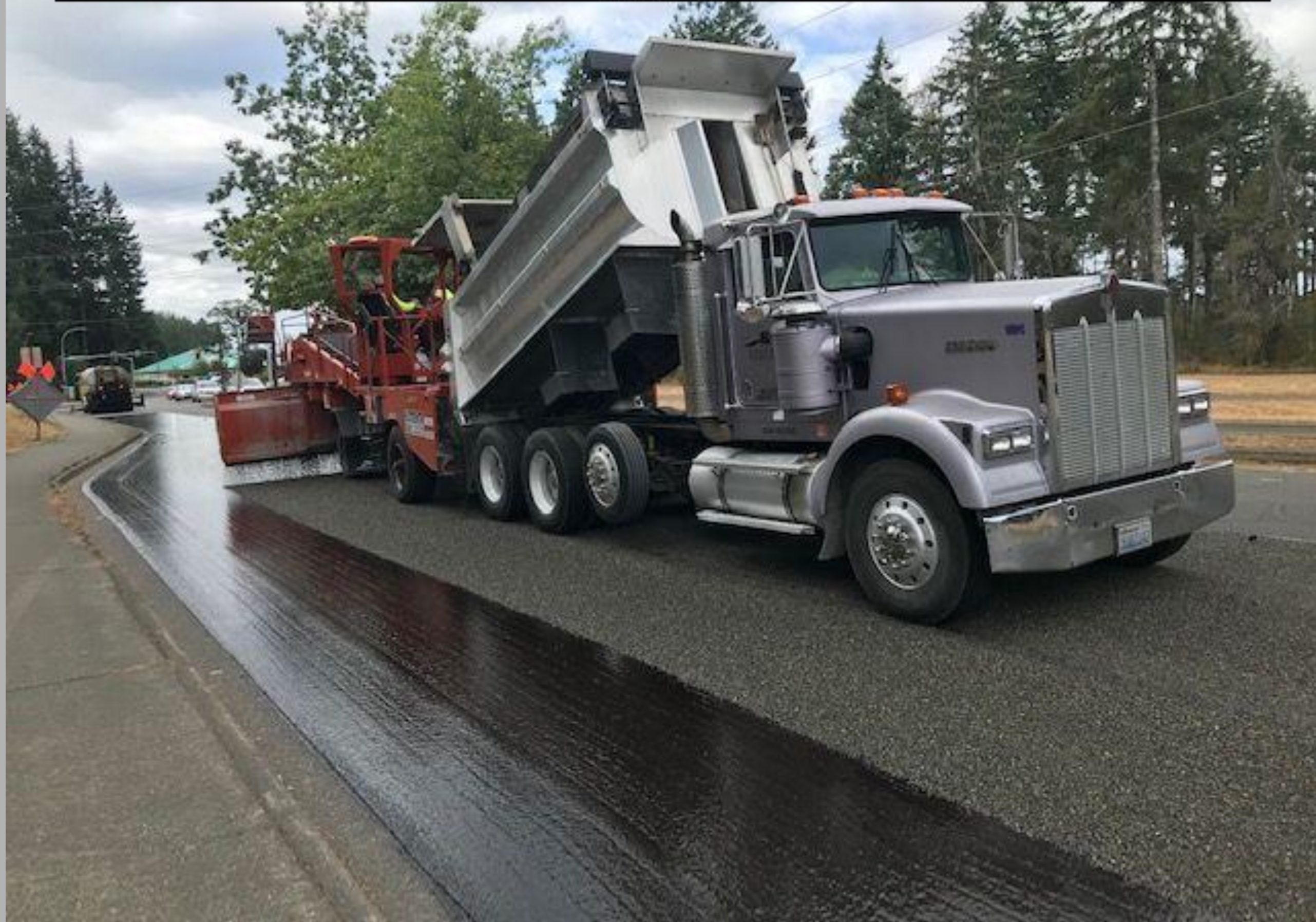
Placing rock on emulsified asphalt in bus stop on N13th infront of Olympic College
