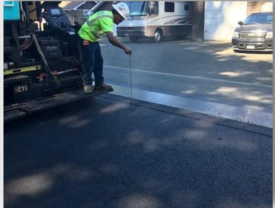
Park Street during 2021 overlay paving
