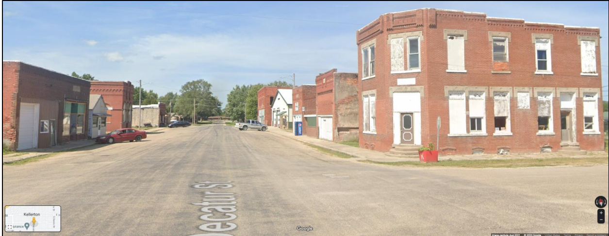
Figure 14. 100 Block of S. Decatur Street in Kellerton, looking north. This commercial area contains brick buildings with a shared historic fabric. There is mixed integrity, and there are few modern infills. This small commercial area may warrant further study. It certainly warrants preservation to some degree. The Odd Fellows Hall (east side north end) was identified by the commission as one of its early interests. Source: August 2021 Google Street View.
