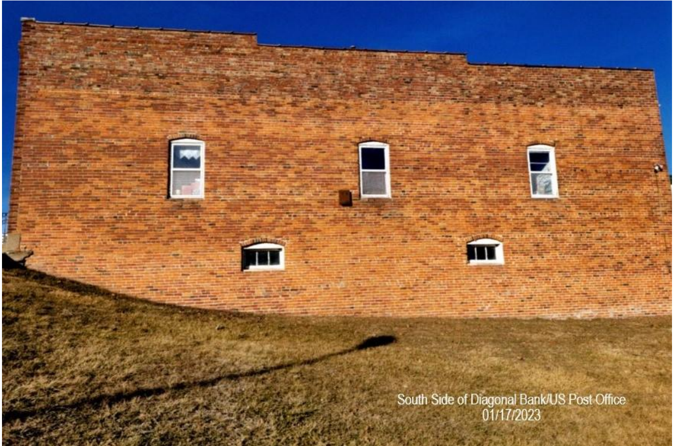
South side of attached post office building, looking north. 01/17/2023.
