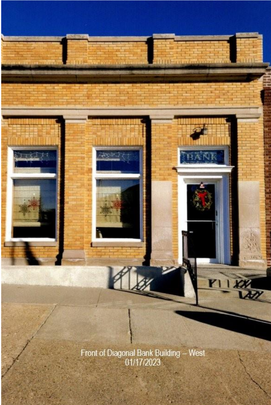
West-facing façade of the bank, looking east. 01/17/2023.
