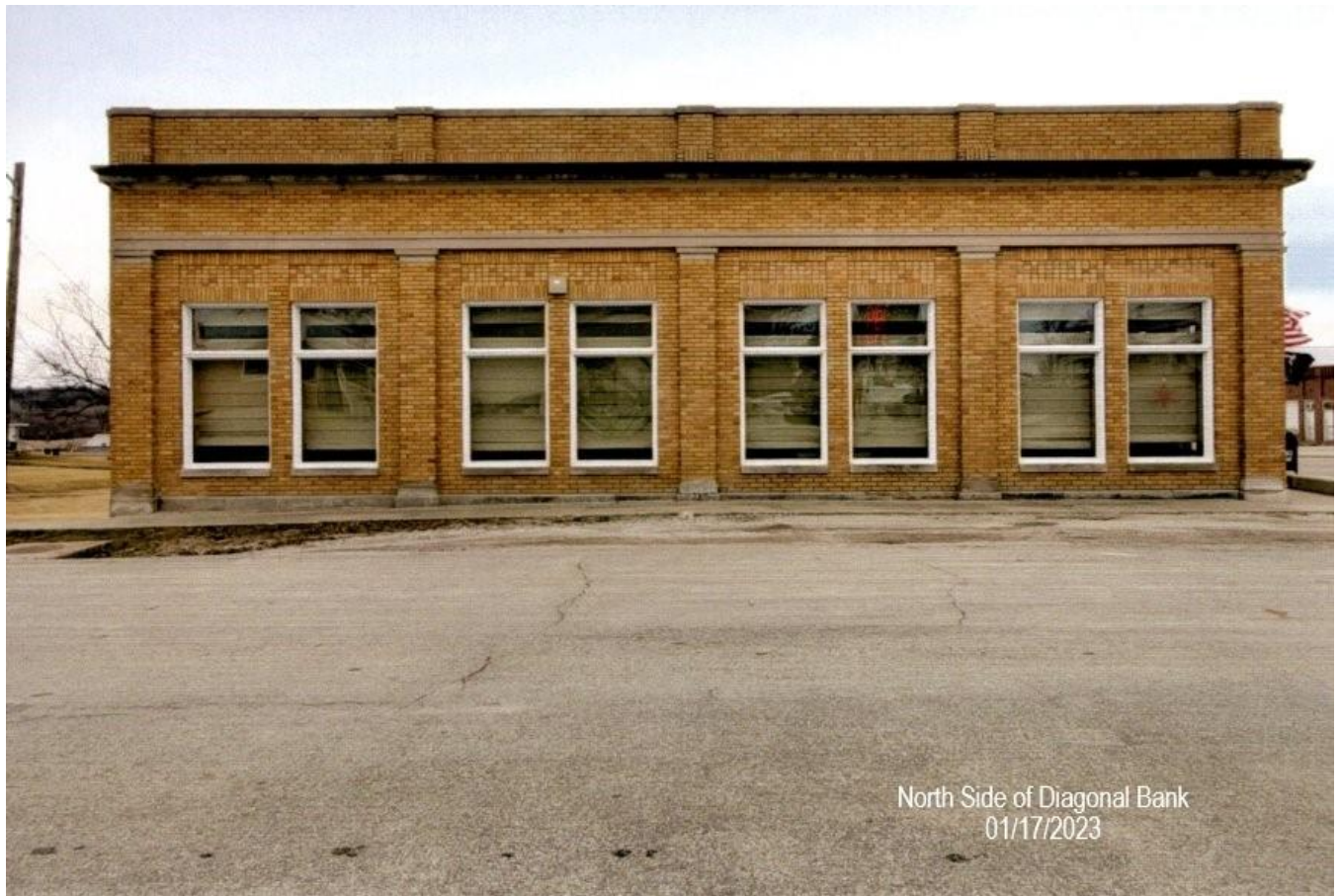
North side of the building, looking south. 01/17/2023.
