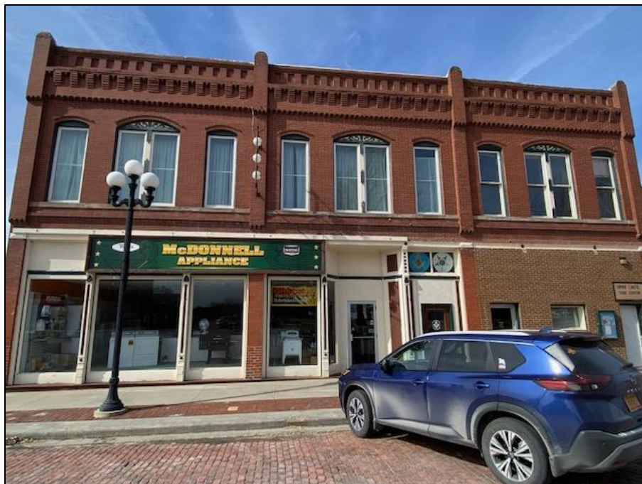
Figure 12. 119-123 S. Fillmore Street, Mount Ayr, looking west. This row of brick commercial buildings may be found to be contributing to a district if given further study. It appears to demonstrate architectural design for Criterion C and may prove to also hold significance under Criterion A and/or B. Photo Source: Korbie Rinehart, February 2023.
