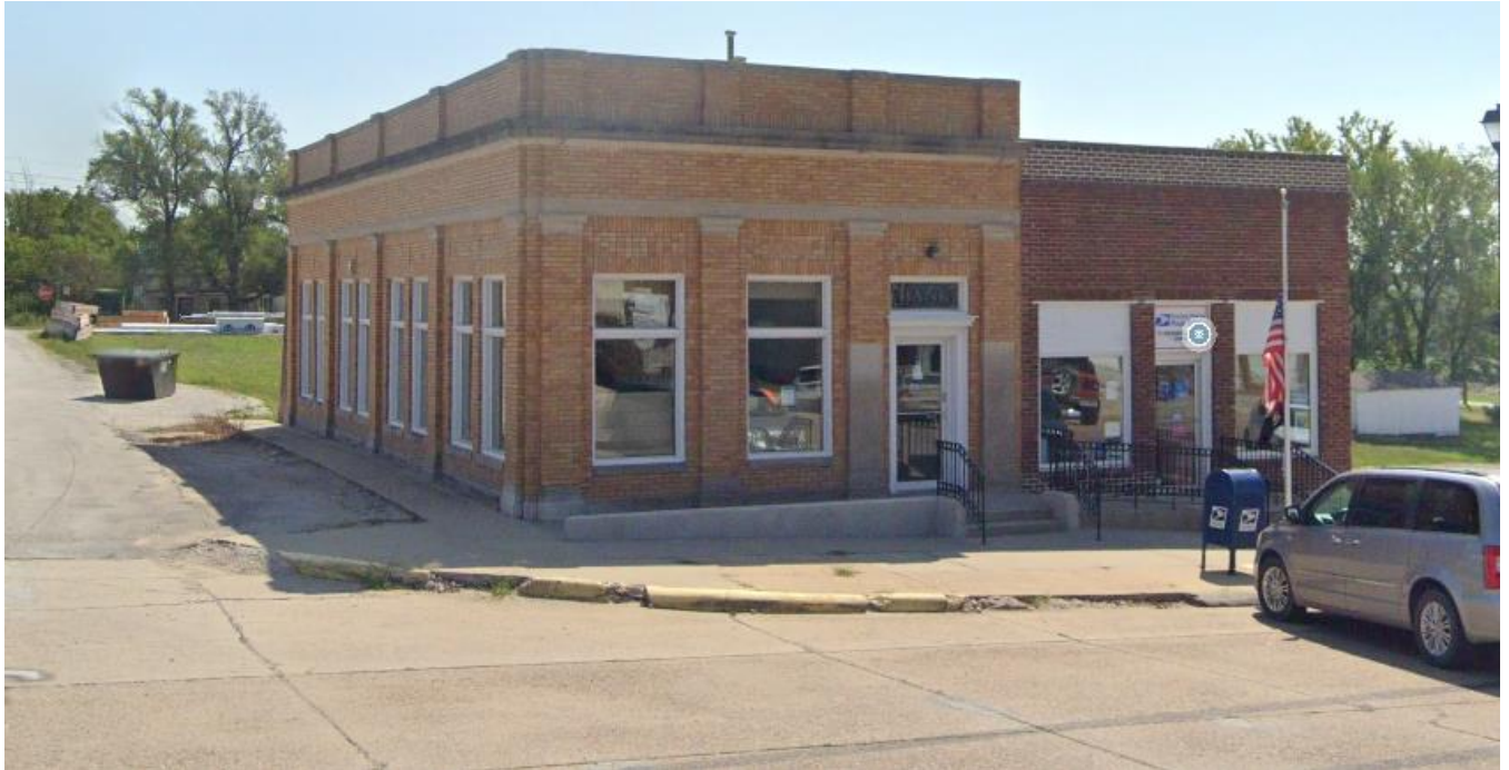
North side and west sides of both buildings, looking southeast. August 2021 Google Street View.
