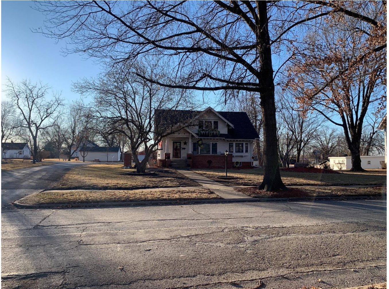
109 Shellway Dr, looking west. Photo: Abby Elliott, March 2023.
