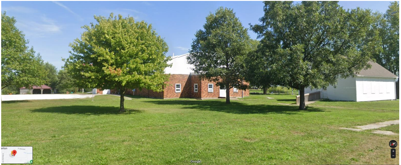
August 2021 Google Street View of the west sides of the community center and museum, looking southeast.
