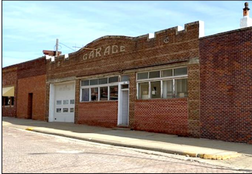
Figure 8. Garage building near the Mount Ayr Square, looking northeast: an example of an automotive garage building, looking northeast, that lies within the potential commercial district outlined later within this document. It may be found to represent the historical context of commerce in the county and city, but it may also represent the history of automobiles' impact on the cultural landscape (all Criterion A). This building has an intricate parapet with text and imagery, it also retains much of its brick exterior materials. Though some of the garage doors have been modified, it very well may still be contributing to this district with additional significance under Criterion C. Photo Source: Korbie Rinehart, February 2023.
