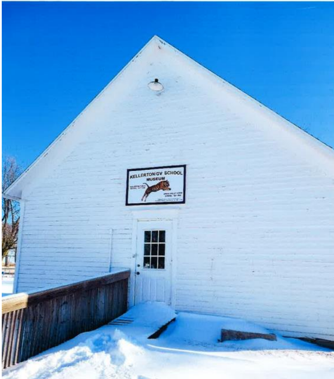
North side of the school museum, looking south. Photo Source: Marlene Tull, January 2023.
