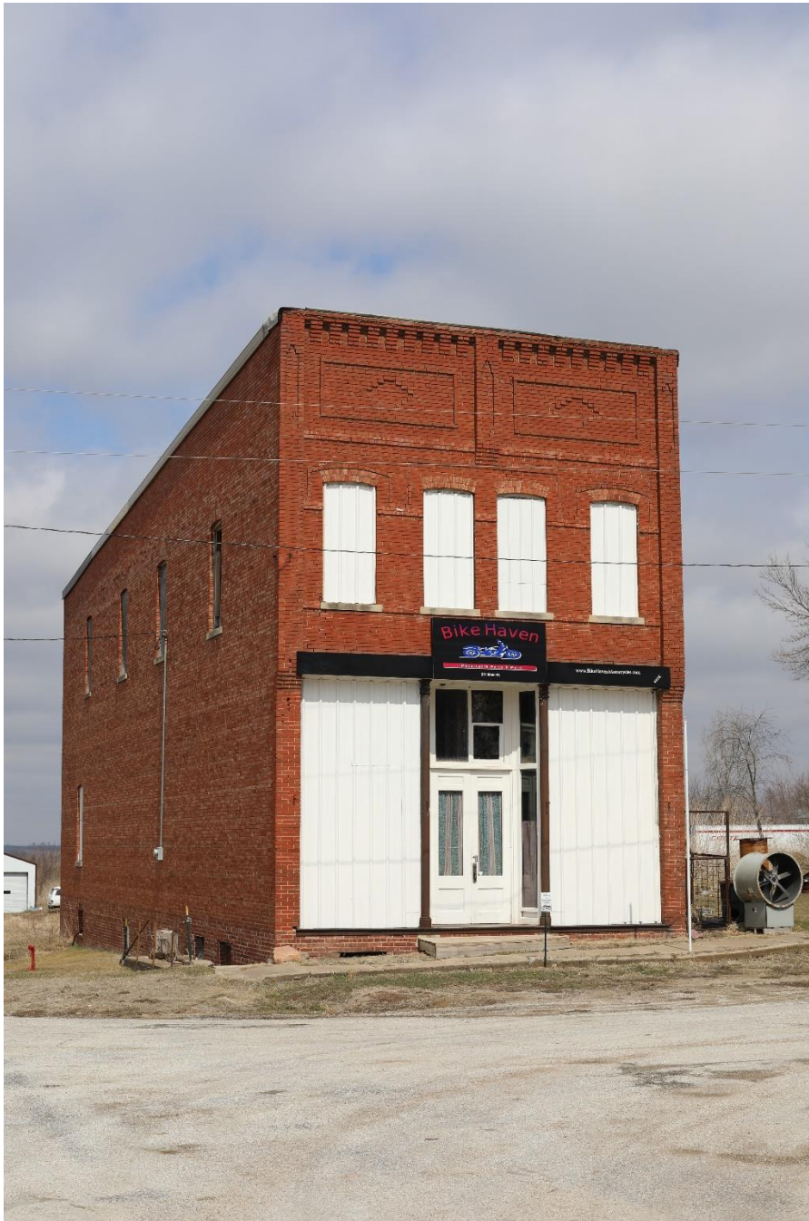
South-facing façade of the building, looking north. Photo: Kim Scharfenkamp, March 2023.
