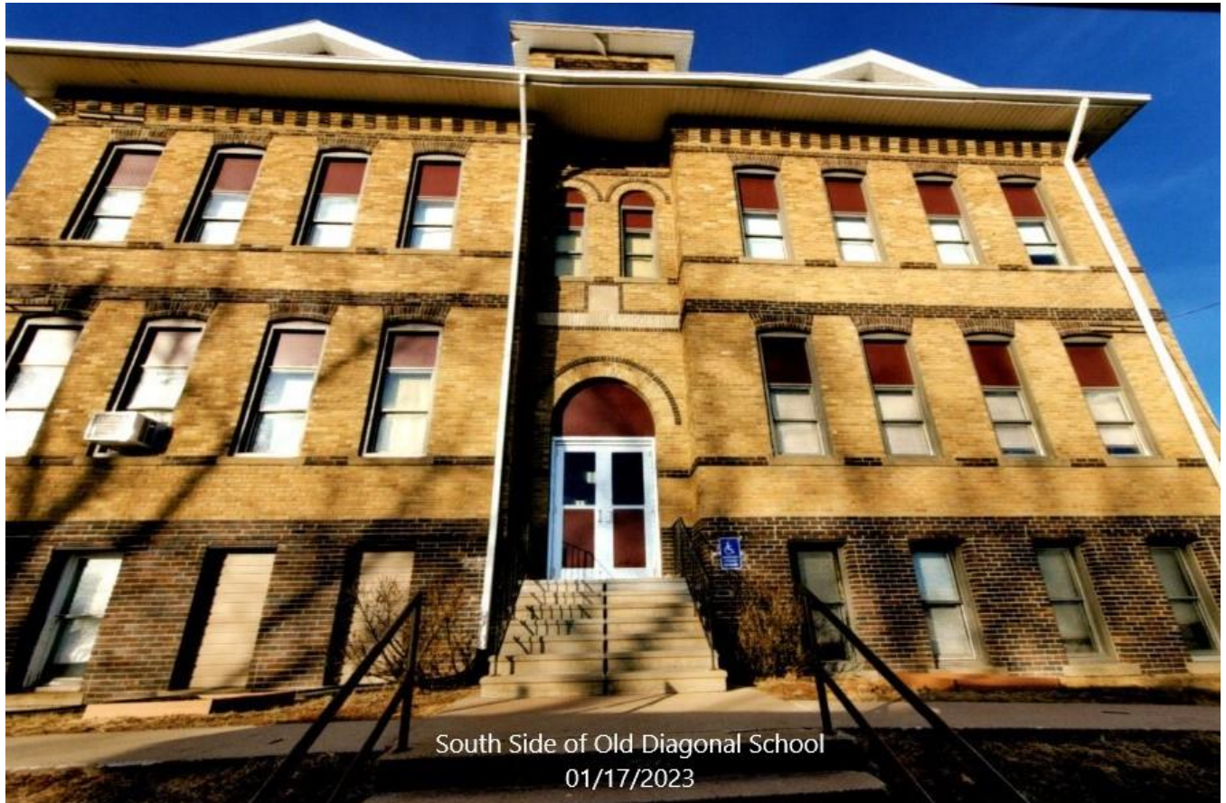
South-facing façade of school building, looking north. January 2023.
