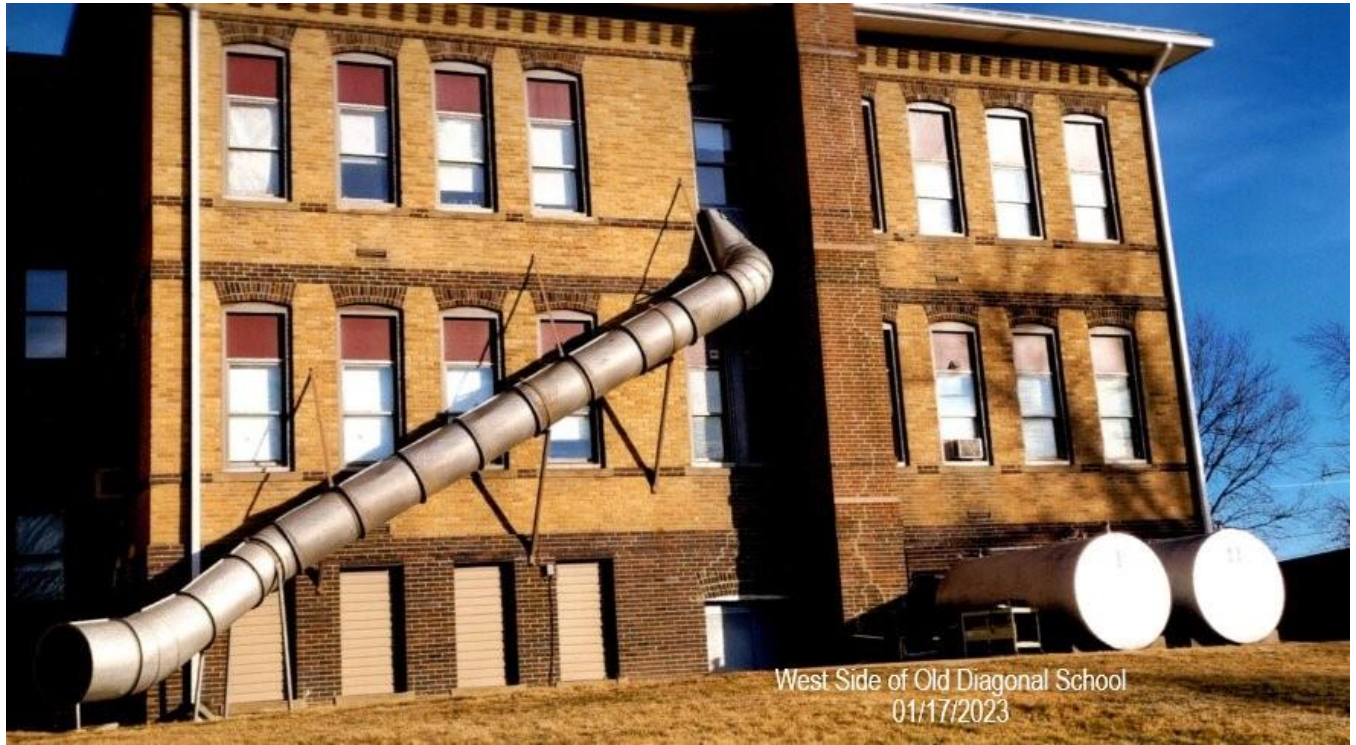
West side of main school building, looking southeast. January 2023.
