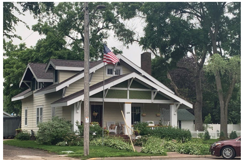
Statz House, built 1921.
