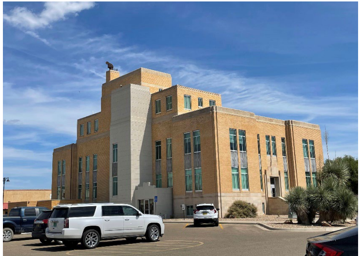
Figure 46 Roosevelt County Courthouse
