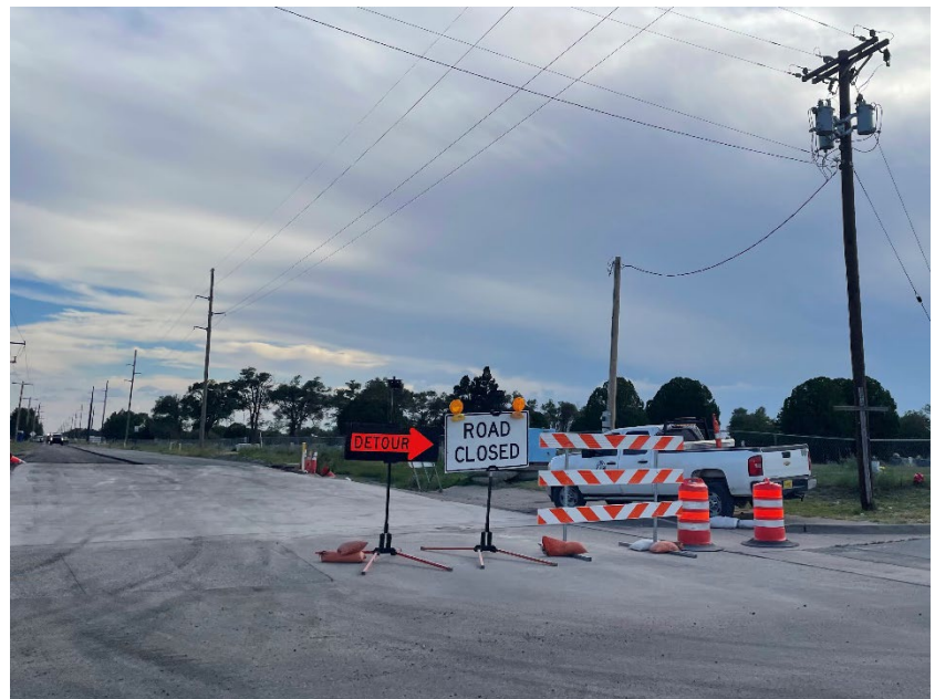
Figure 47: Road resurfacing on Kilgore Avenue
