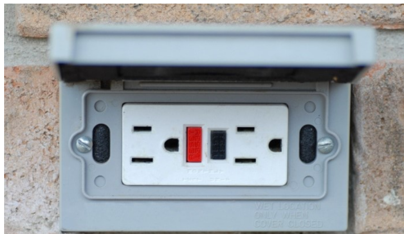
GFCI protected exterior outlet
