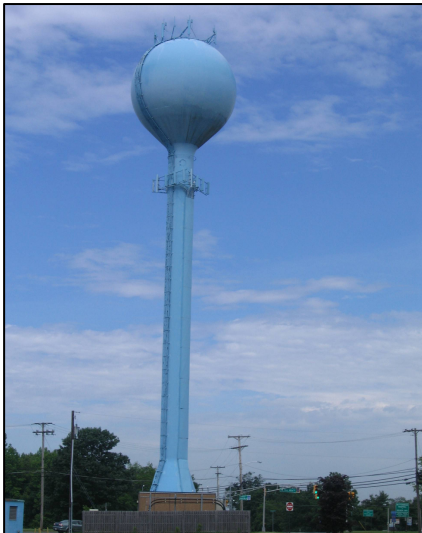
Water tower at the intersection of Pemberton Browns Mills Road and Four Mile Road
