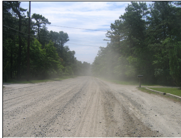
Dust generated from car traffic on North Whitesbog Road impacts residential homes
