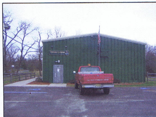
D. Johnson Recreation Center
