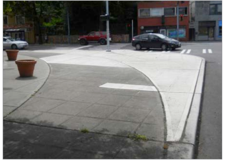
This modified curb radius reduces the speed of turning vehicles and shortens the pedestrian crossing. (Credit: Michael Hintze/pedbikesafe.org)
