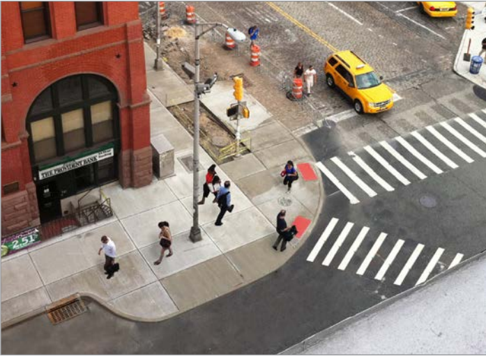
A constructed curb extension improves pedestrian conditions at this busy intersection in Hoboken, NJ
