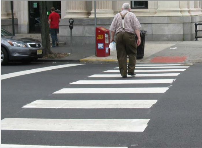
High-visibility crosswalks have been shown to increase motorist yielding and channelization of pedestrians.
