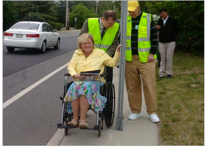
Good planning can help avoid the situation pictured here and maintain pedestrian facilities with appropriate clear zones, free of obstacles, such as sign posts or utility poles.
