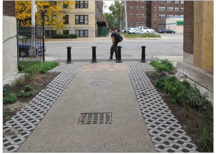
Permeable pavements and rain gardens help absorb and infiltrate stormwater (Source: NACTO)
