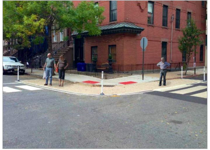
A painted (epoxy) curb extension with pylons is an effective interim or low-cost solution
