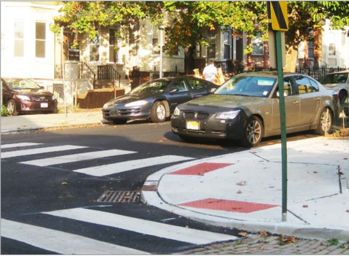
Intersections should have two perpendicular, ADA compliant curb ramps per corner, as shown in this example from Jersey City, NJ.
