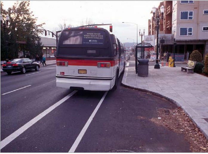
A “bus bumpout” is an extension of the sidewalk that enables safe and efficient access between the sidewalk and the bus. (Source: pedbikeimages.org)
