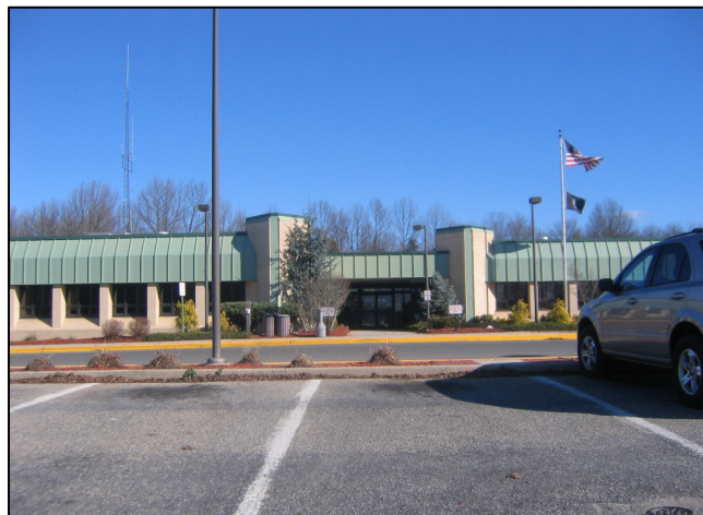
Pemberton Township Municipal Building
