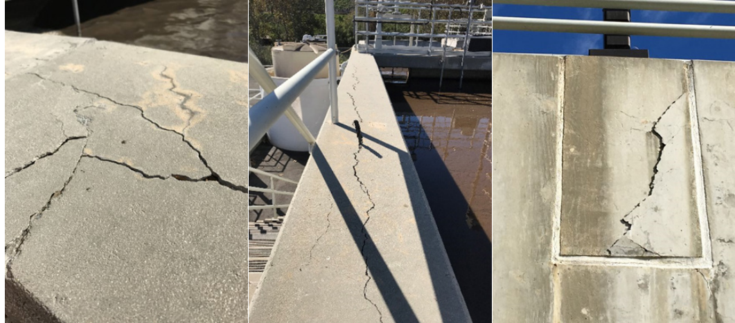
Figure 6 Examples of Cracks Visible in the Ditch No. 1 Structure
