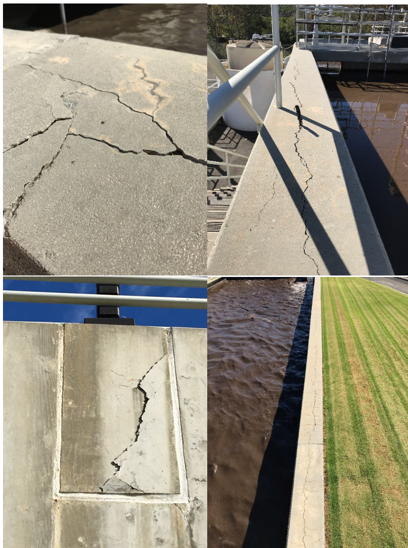
Figure 6.5 Cracks in the Oxidation Ditch Structure - Ditch No. 1
