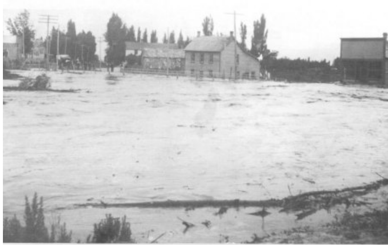
Looking south, the water flooded streets and filled basements in the lower end of town
