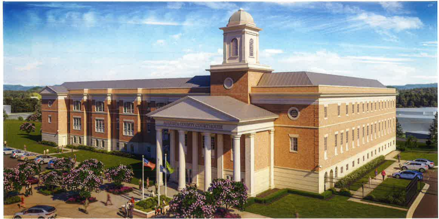
ABOVE Following our space needs assessment and master plan for the Augusta County courts system, our team developed designs to relocate the county's courthouse functions to a new 123,373-square-foot courts complex.
