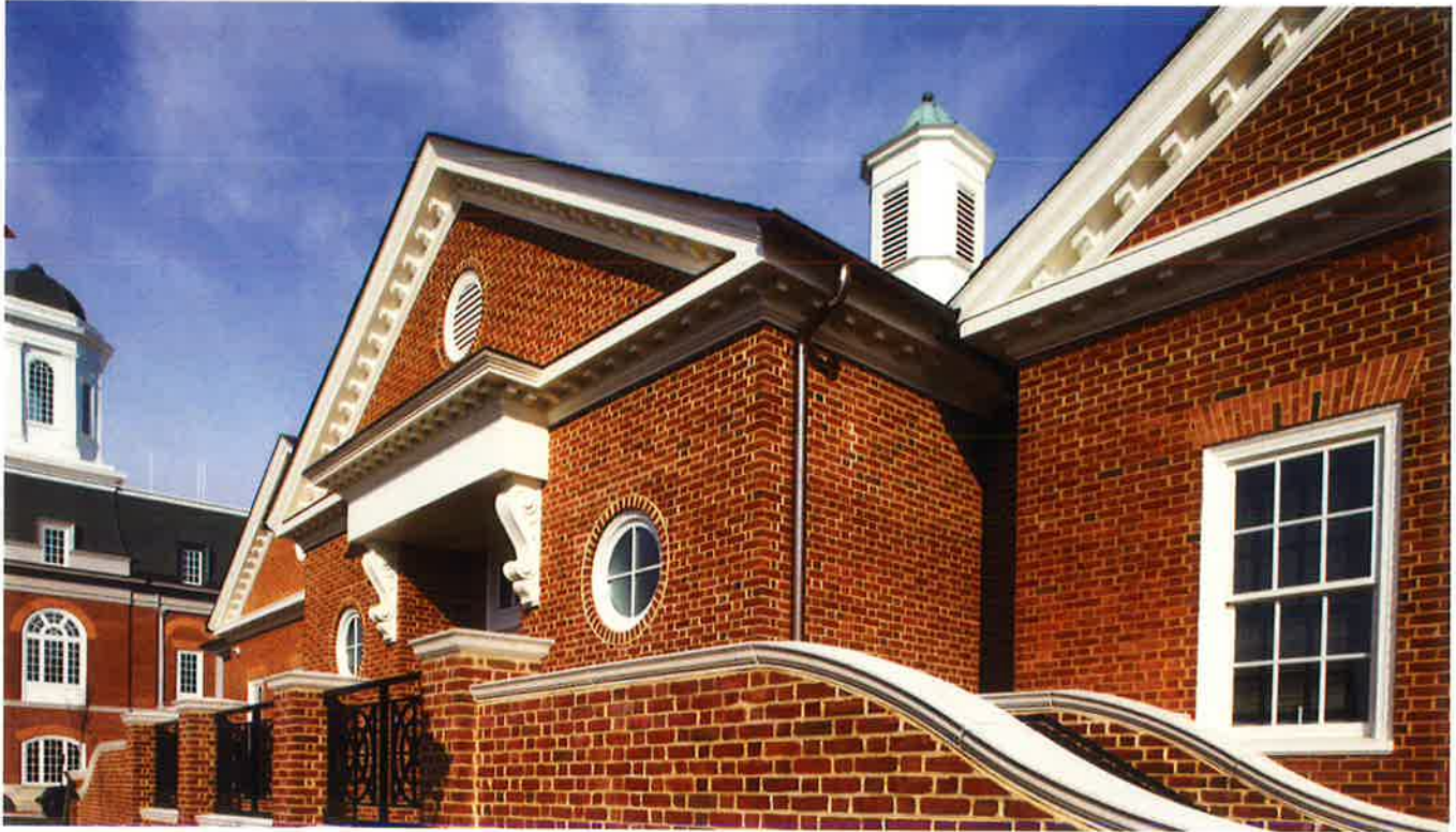
ABOVE Juvenile and Domestic Relations Court Renovation, City of Fredericksburg
