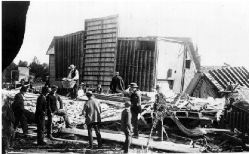
Residents clear tornado damage near the old water works after the May 1896 storm (photo donated by Henk Photography)
