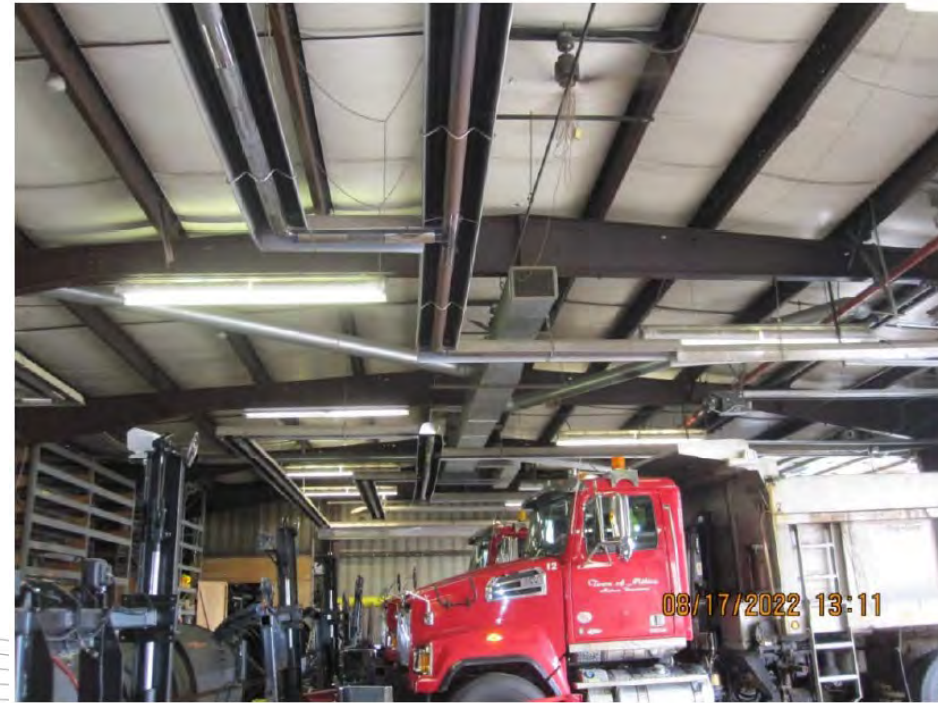
Photo 7 – Abandoned Infrared Heating & Exhaust Fan – Looking South
