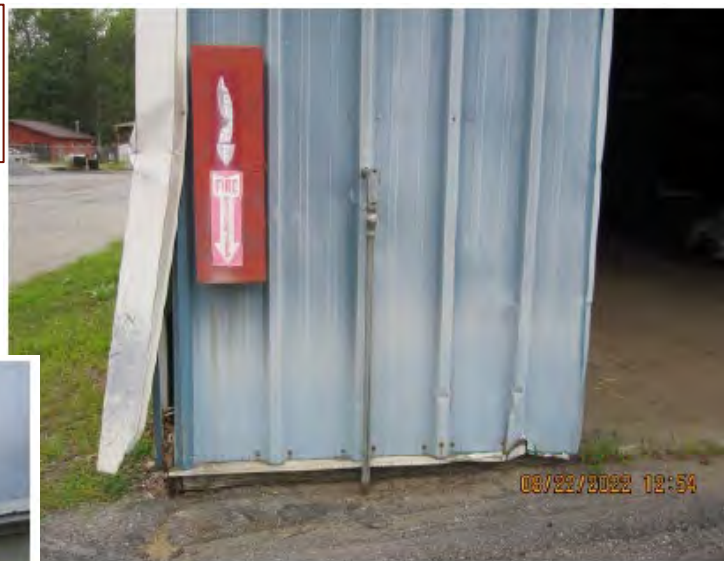
Photo 5 – Damage to Metal Siding and Trim, Looking West
