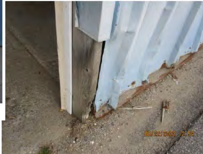
Photo 6 – Damage to Metal Siding and Jamb, Looking Northwest
