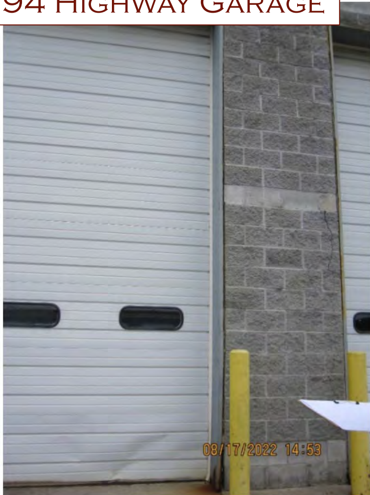
Photo 3 – Crack in Exterior Masonry Wall, Looking East
