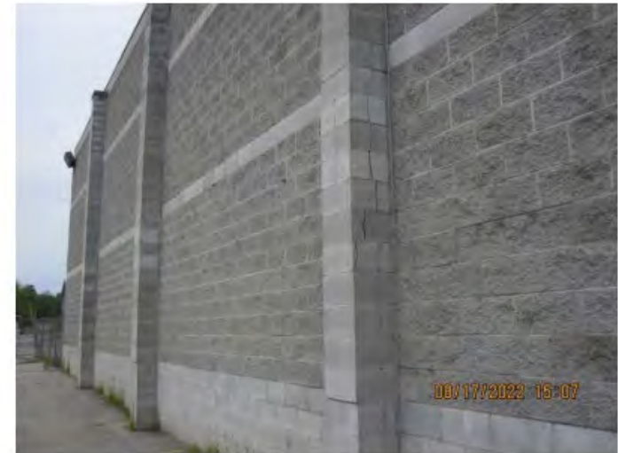
Photo 11 – Cracks at Exterior Masonry Pilasters, Looking Northwest
