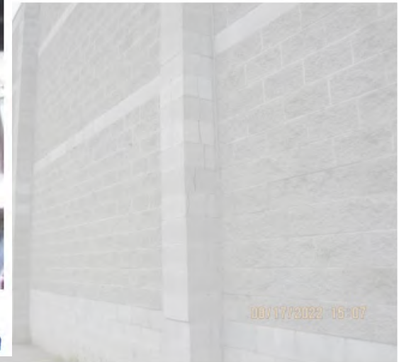
Photo 11 – Cracks at Exterior Masonry Pilasters, Looking Northwest
