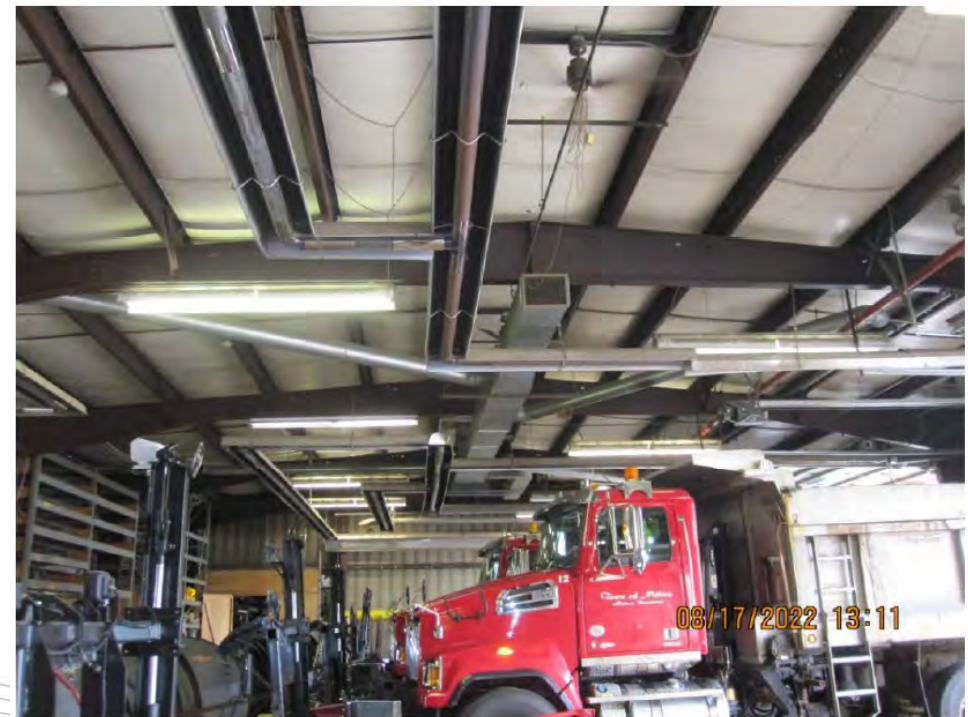
Photo 7 – Abandoned Infrared Heating & Exhaust Fan – Looking South
