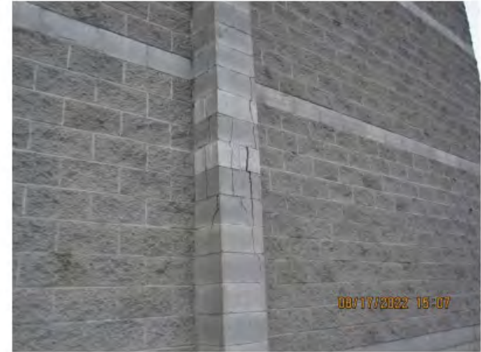
Photo 10 – Cracks at Exterior Masonry Pilasters, Looking North
