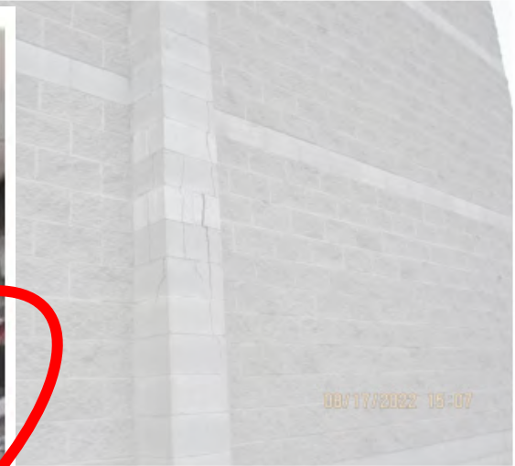
- Cracks at Exterior Masonry Pilasters, Looking North
