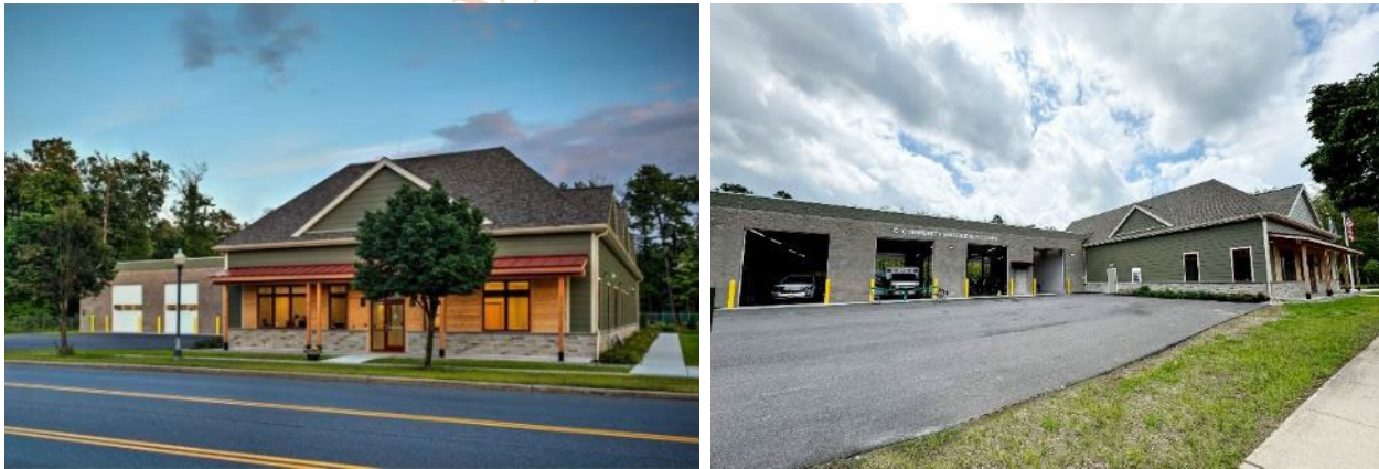
(Above) New Community Ambulance Corp Facility, Ballston Spa
