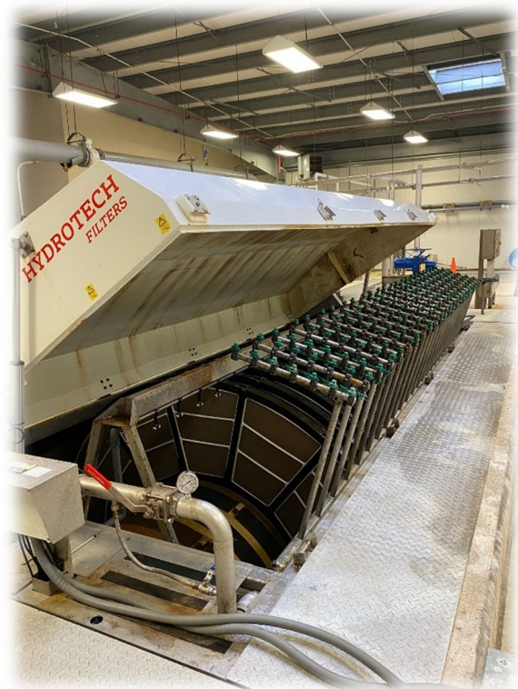
Disk Filters at WWTP.
