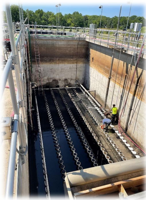
Cleaning and inspection of SBR Basin
