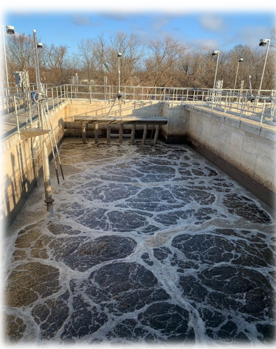
Operational SBR Basin at WWTP
