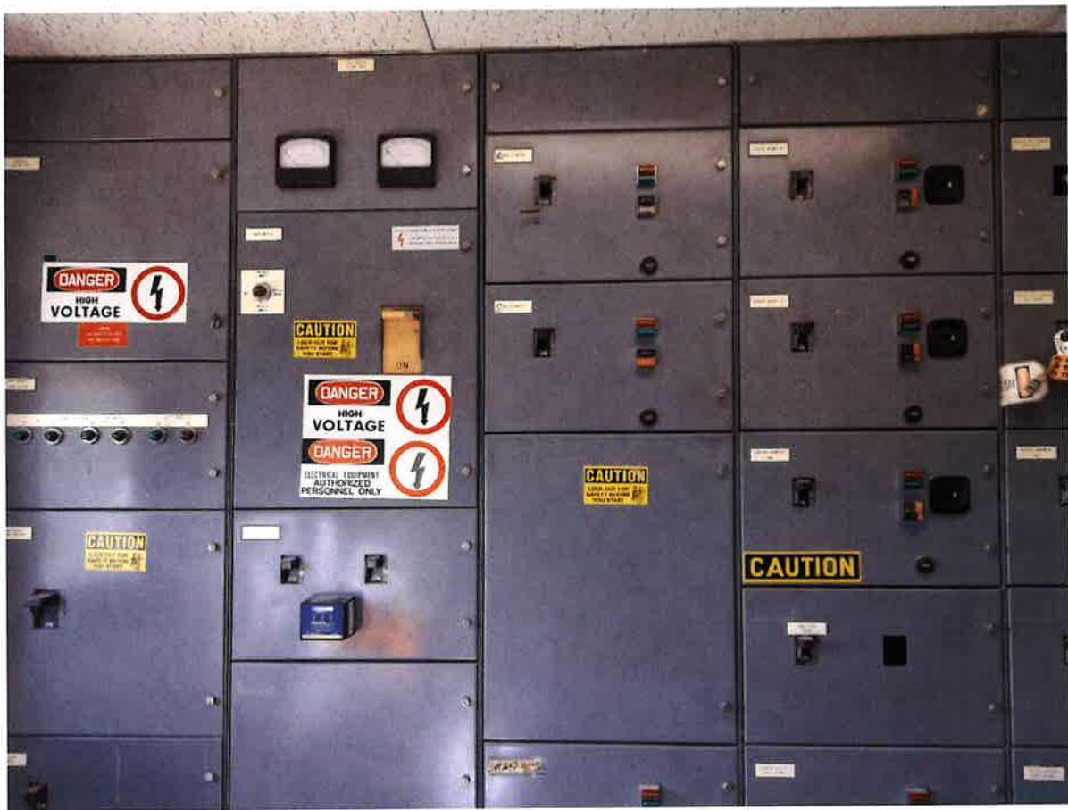
West Plant Motor Control Center
