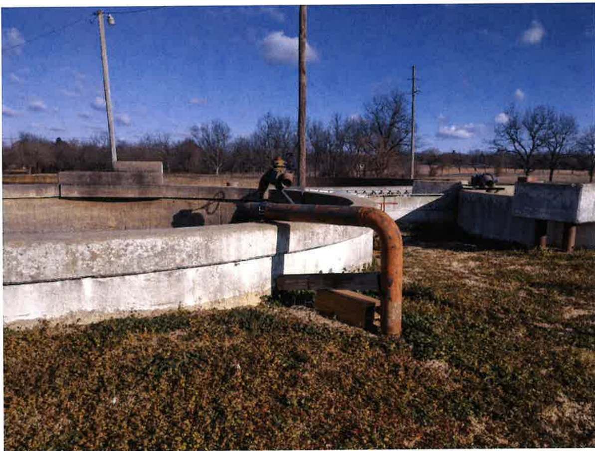
Air Piping into West Digester at East Plant
