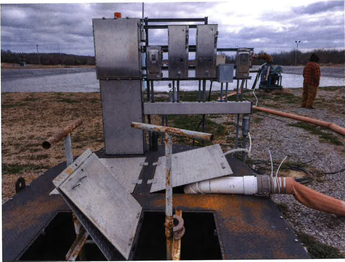
Pump Station Out of 9 Million Gallon Flow Equalization Basin At East Plant. Original Suction Pipe blocked. Operators Set Up Semi Permanent Hoses for Flow Out of Basin.
