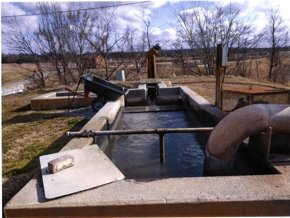
Grit Basin at East Plant. Equipment for Grit Removal Has Not Functioned For Many Years.
