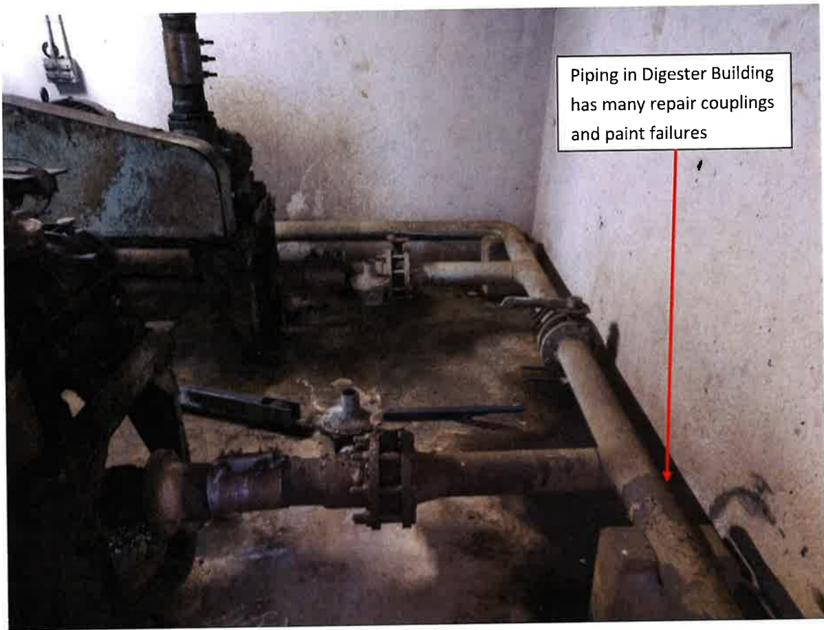
Air Piping and Blowers (to left) in Digester Building at West Plant
