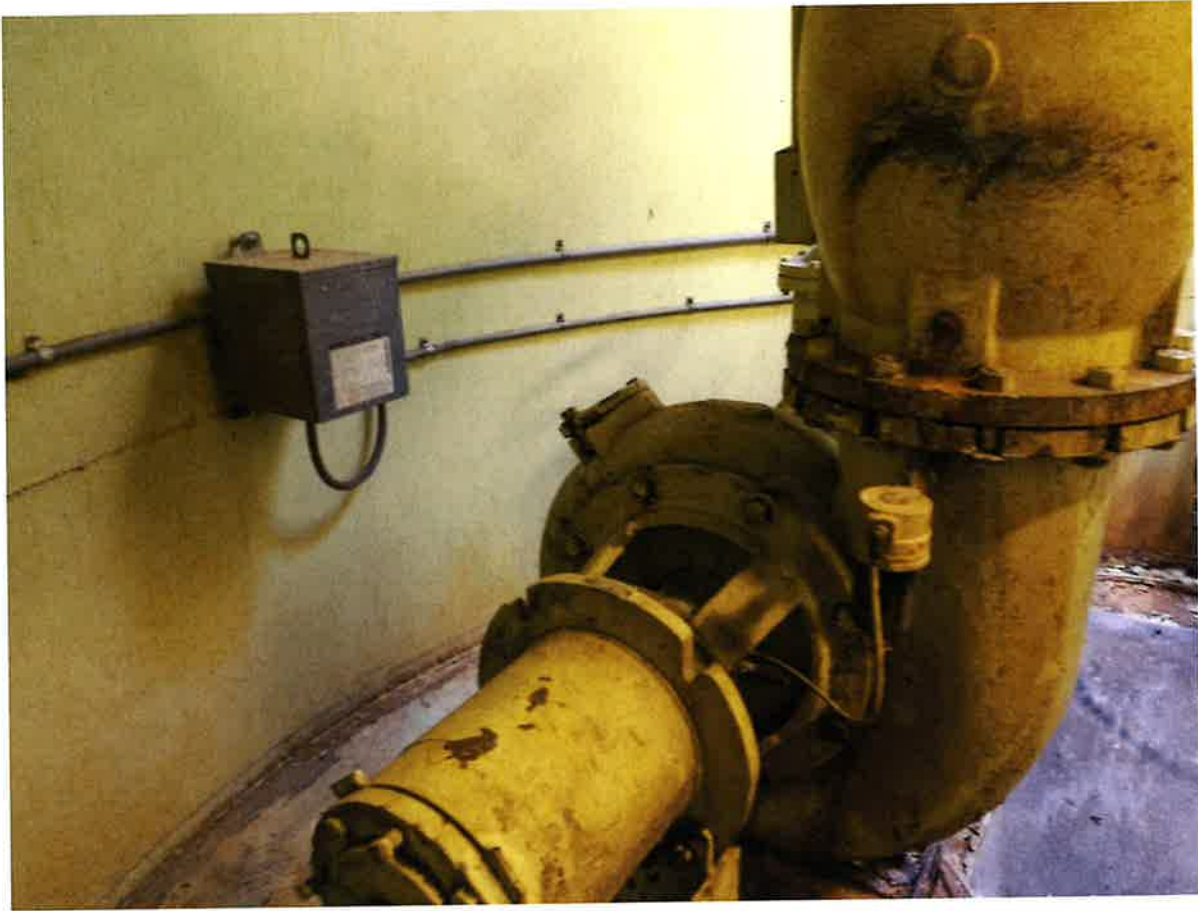
Stormwater Pump at East Plant
