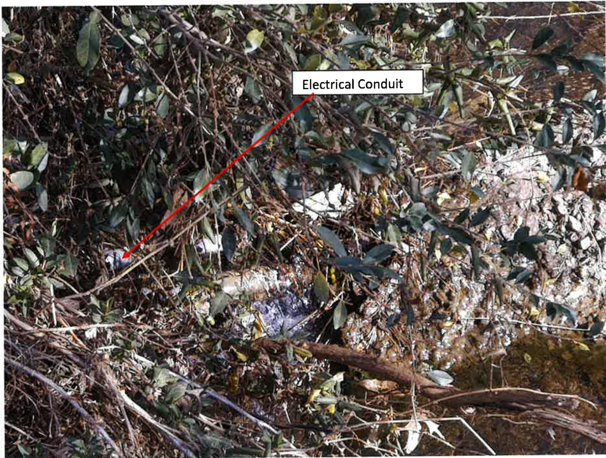
Electrical Conduit at Bottom of Creek at East Plant
