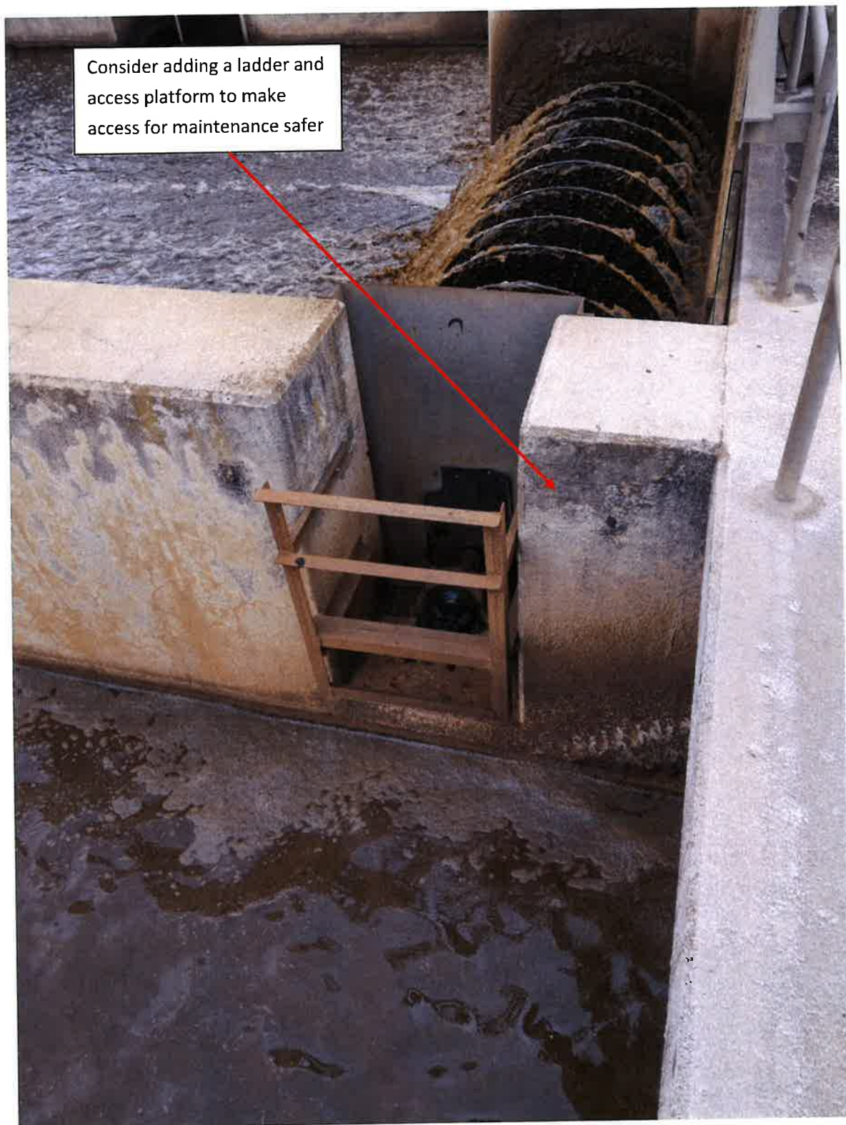
View of aerator bearing that operators must access for maintenance
