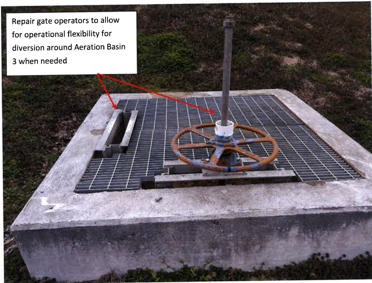
Flow Diversion Box at West Plant Aeration Basin 3
