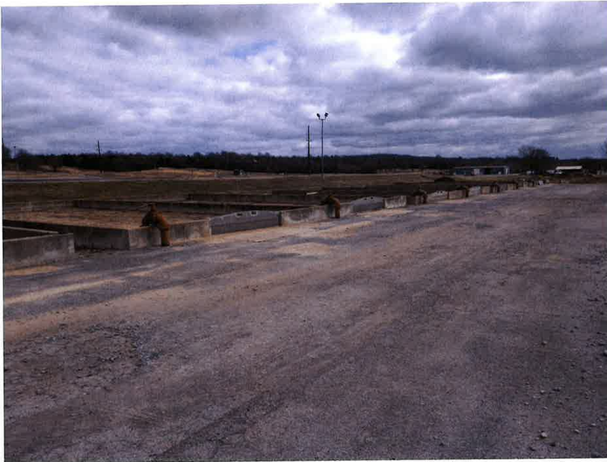
Drying Beds at East Plant
