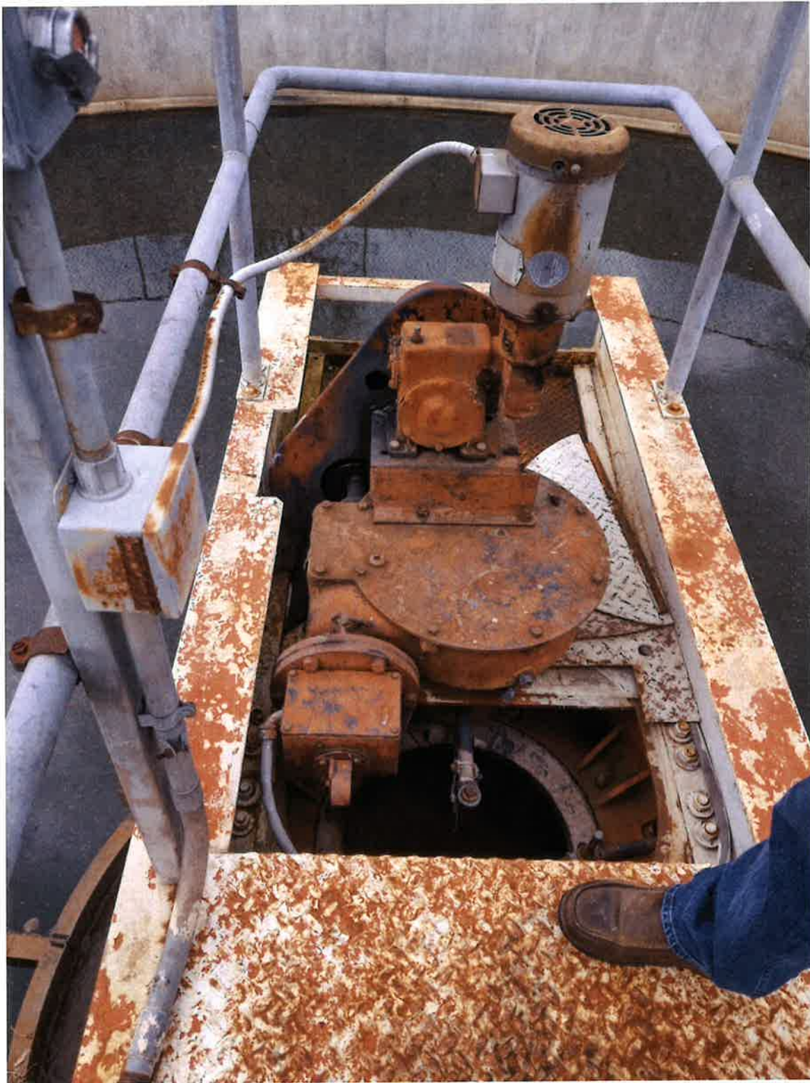
North Clarifier Gear Box and Motor
