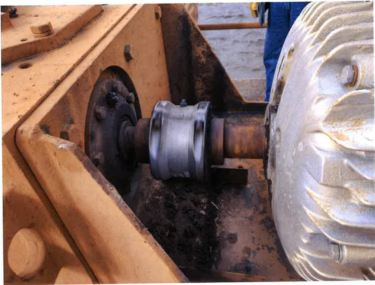
Motor to Aerator Coupling Missing Safety Guard
