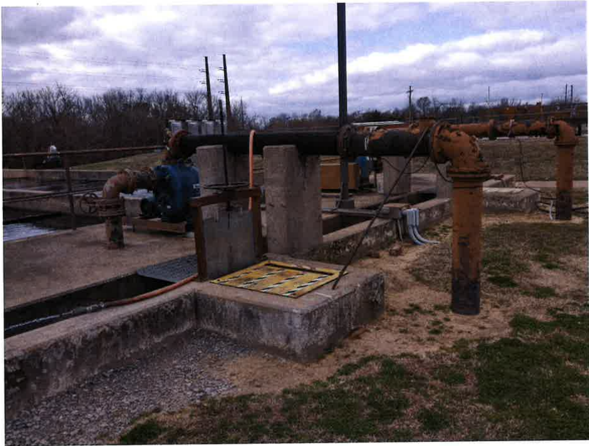
RAS Pumps at Final Clarifiers at East Plant
