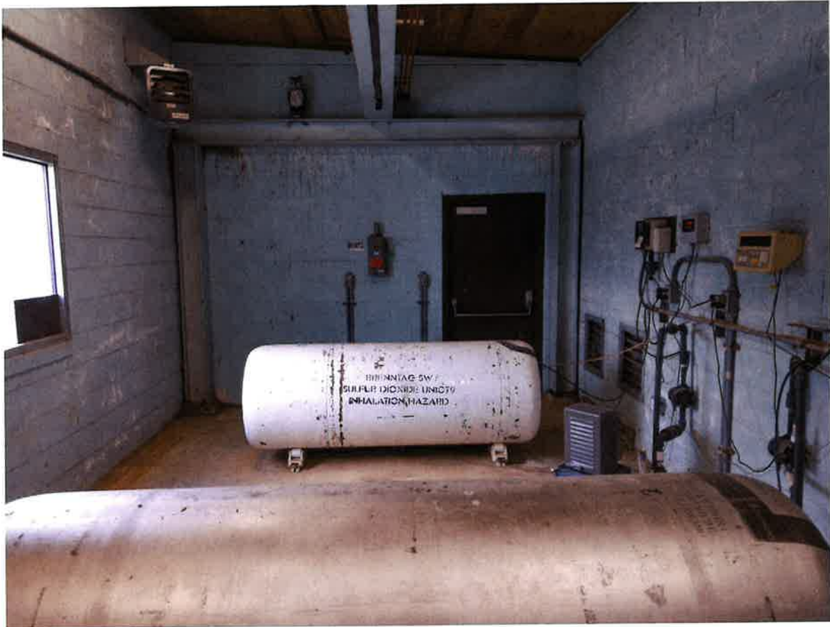
East Plant Chlorine Building. Chlorine Cylinder in foreground, Sulfur Dioxide Cylinder in Background.
