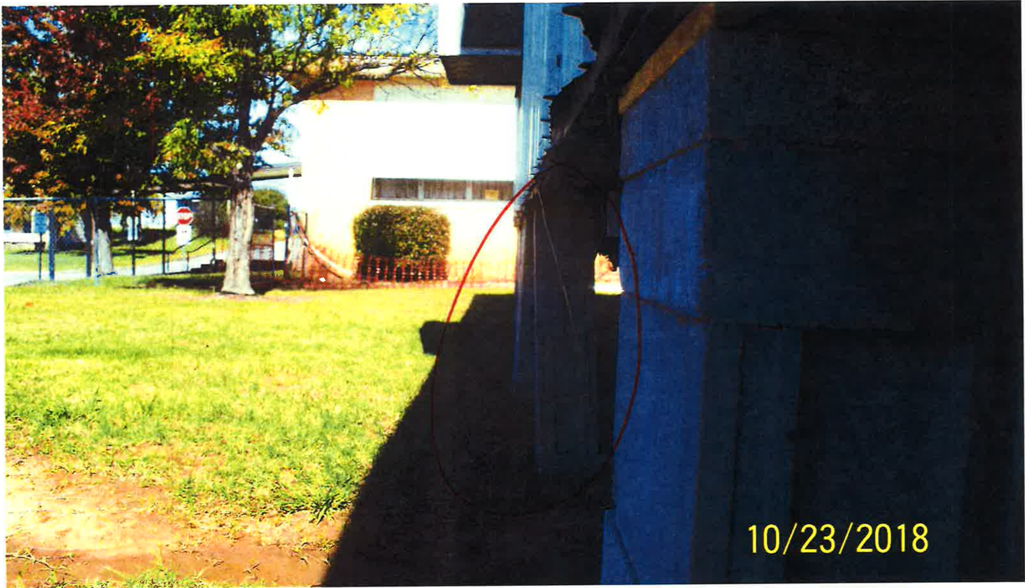
Cinder Blocks leaning because not on proper foundation
