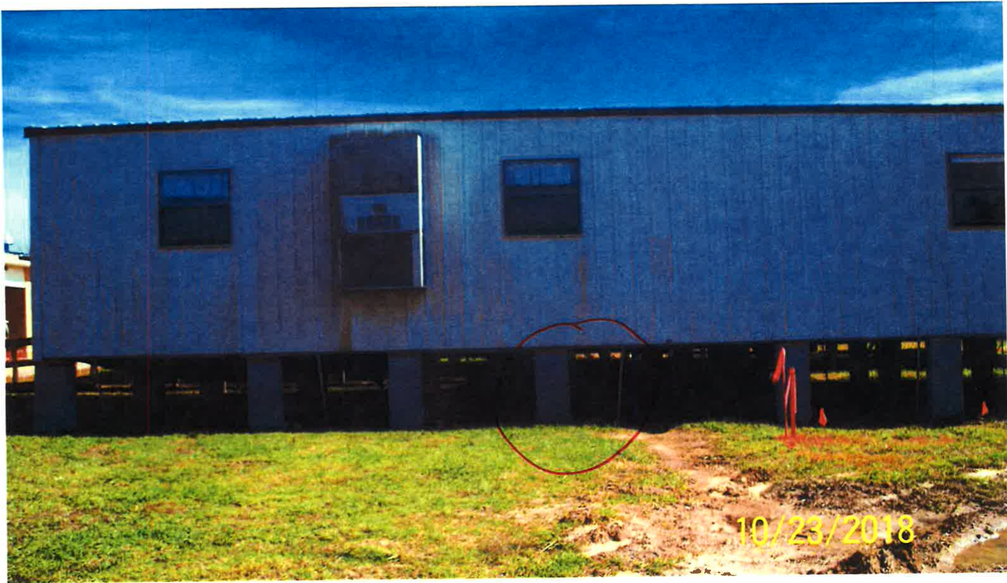
Blocks leaning, no proper foundation
