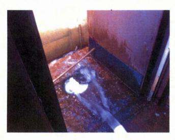
The control valves on each of the four high service pumps have abnormally high leakage. See photograph at left illustrating the volume of water leaking through the valves. In addition to the header pipe replacement, the City should include in this scope of work the rehabilitation of the control valves to reduce excessive leakage.
