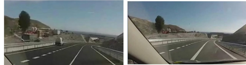
Figure 38: Wider pavement markings can greatly impact the feel of the road. Note that the above comparison is between 4" markings (left) and 12" markings (right).
