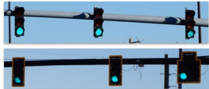
Figure 39: Backplates increase contrast between signal bulbs and the background.
