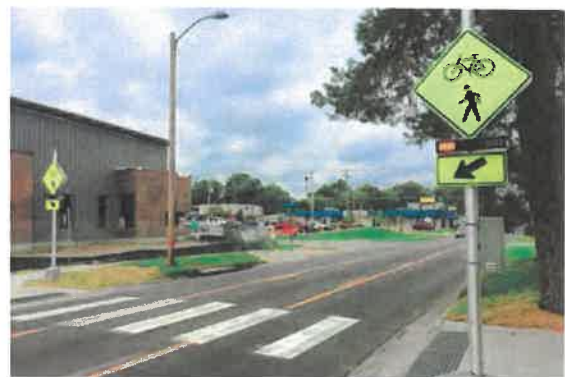
Rectangular Rapid Flashing Beacon (RRFB)
