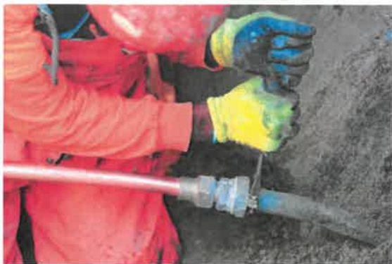
Lead Water Service Line Replacement
