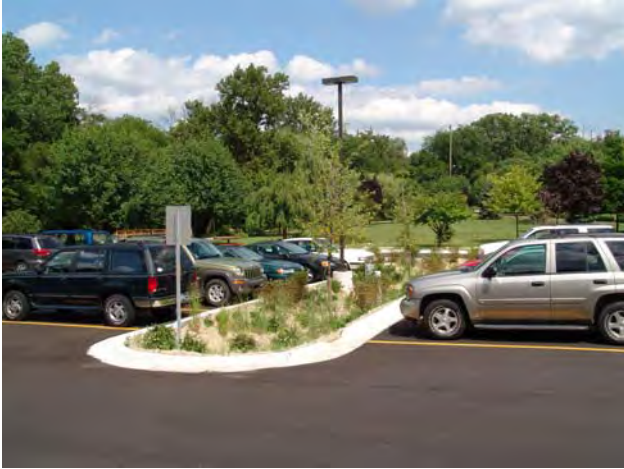
Use of Bioretention within a Parking Lot: Wayne City Hall (Photo courtesy of Alicia Askwith, Ayres Lewis Norris and May)
