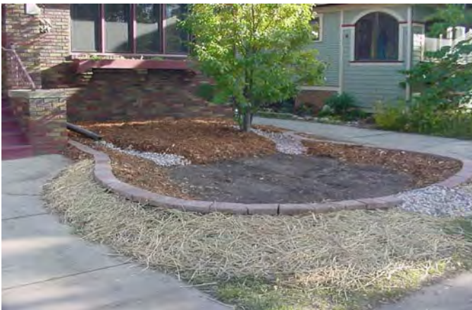
Use of Bioretention within a Residential Development
