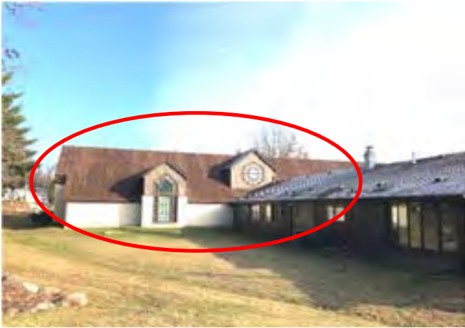
View of the south slope on the west side of the Church
