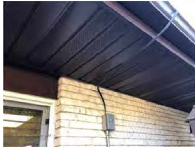
Perforated soffit panel vents.
