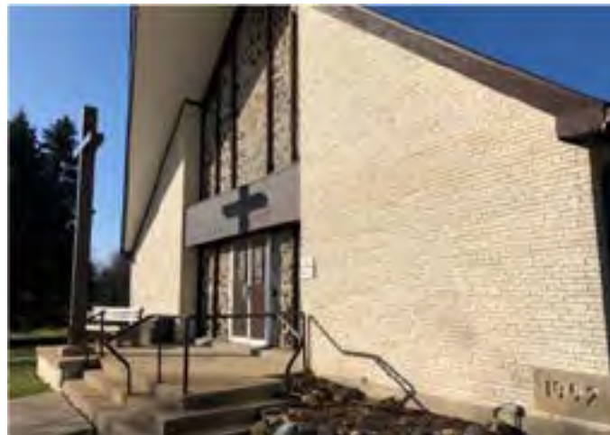
East elevation of Church. Masonry is in good condition.
