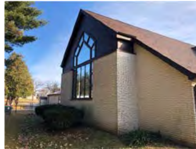
West elevation of the Church.
