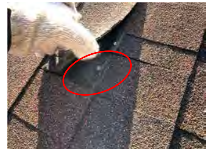
Shingle fastener location.
