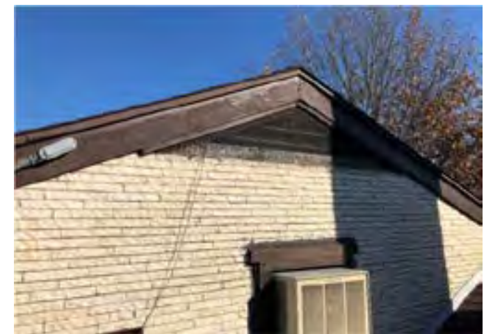
A gable vent was observed over the Parish Center from the roof level.
