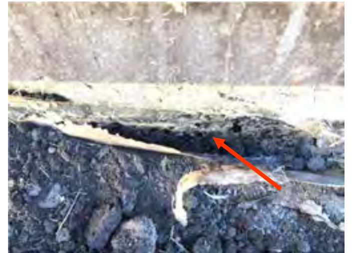
Bituminous water/damp proofing observed at the Rectory/Parish Offices basement foundation wall.
