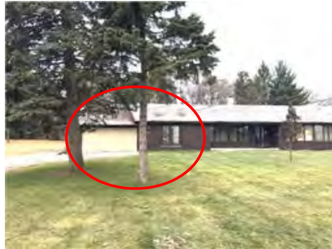
Overview of hot spots on garage and south end of Rectory / Parish Offices
