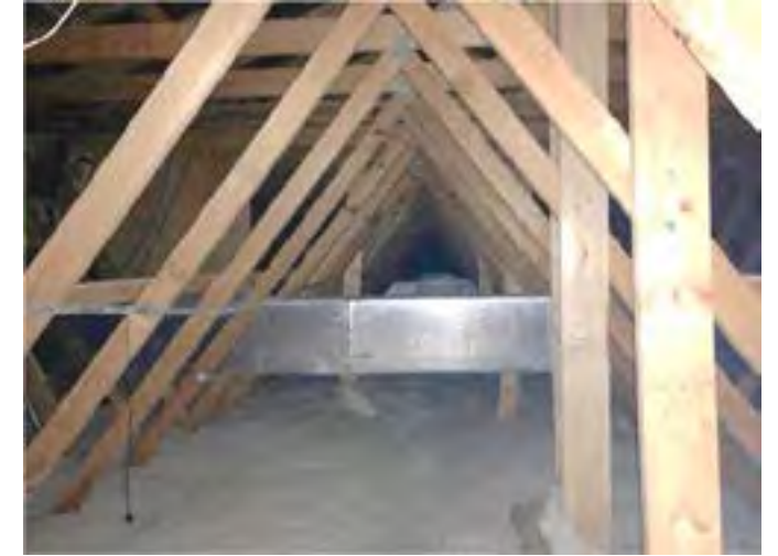
Interior attic space facing north.
