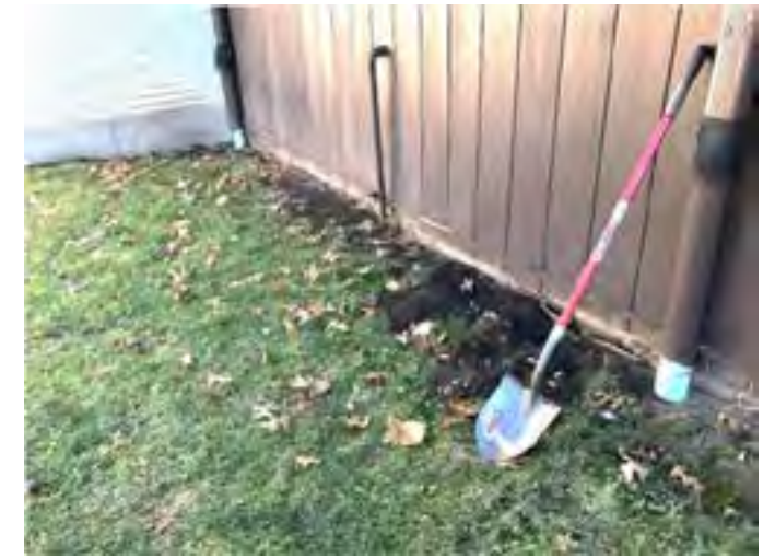
Observation hole next to foundation on west elevation at Rectory/Parish Offices.
