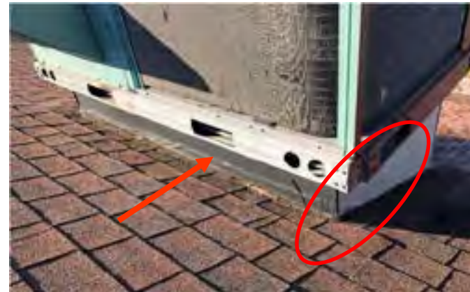
Self-adhered flashing membrane observed on up slope side of HVAC unit.
