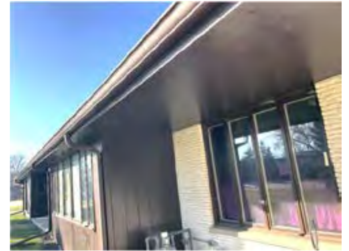
Wood soffit panels were observed.
