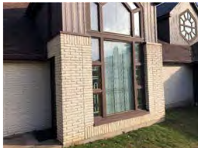
Typical brick veneer condition along south elevation of the Church
