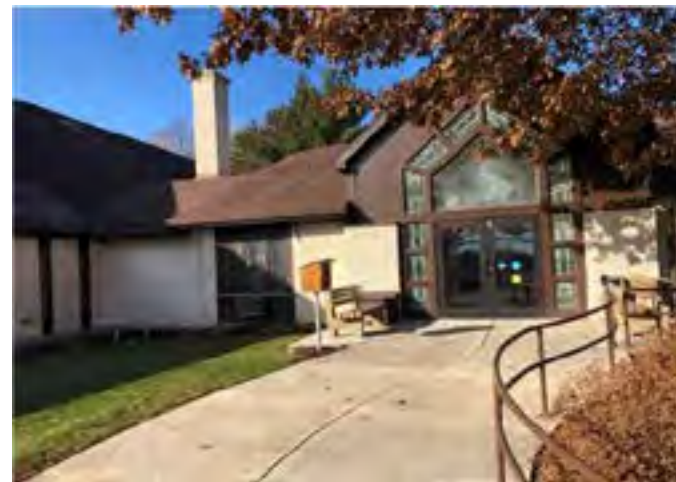
Overview of the exterior of the Narthex area.
