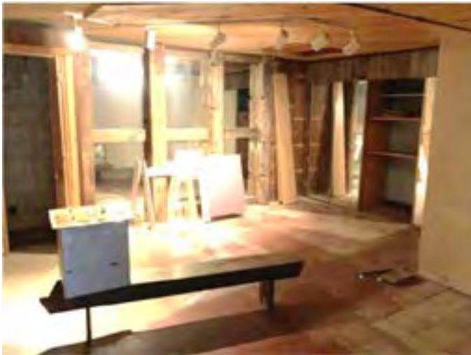
Remediation still underway.
