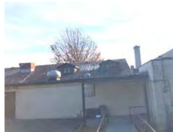
West elevation of the Parish Center at the Narthex.
