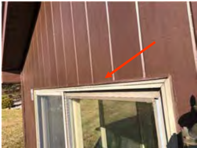
Typical window penetration head condition.
