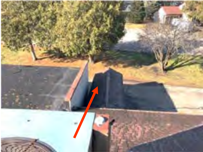
View of lower shed shingle roof.
