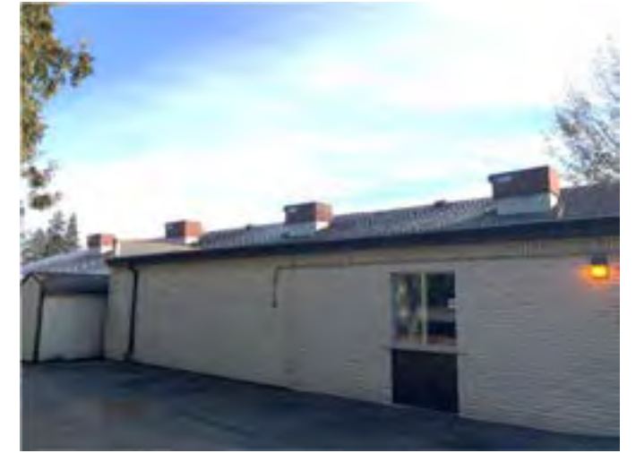
West elevation of the Parish Center.
