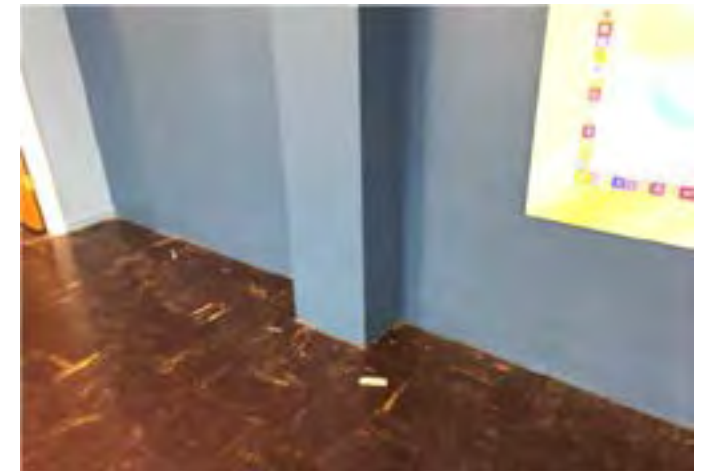
No active leaks observed in the classroom.
