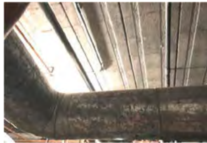
View of hybrid hollow core structural ceiling.
