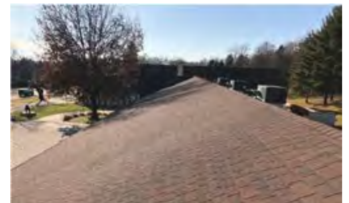
Overview of east slope of the Parish Center facing south.
