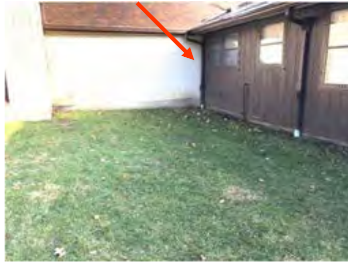
Inside corner where Rectory/Parish Offices meets the Church.
