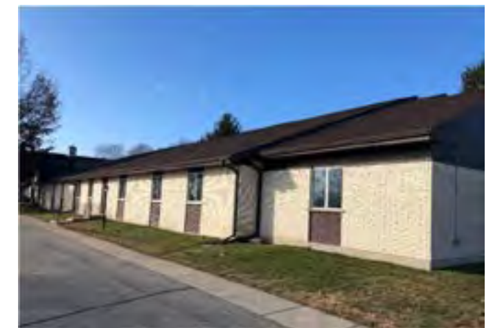
Overview of east elevation of the Parish Center facing southwest.
