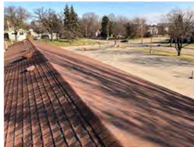
Overview of east roof slope facing north
