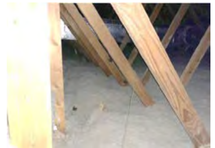
Interior of attic space facing northeast.
