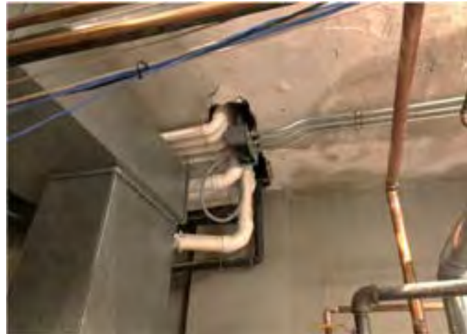
PVC pipe penetrations through mechanical room ceiling. No active leaks observed.
