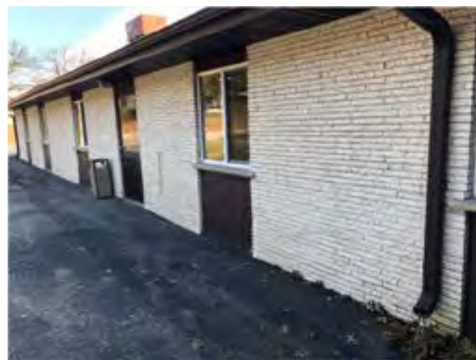
Overview of west elevation of the Parish Center.
