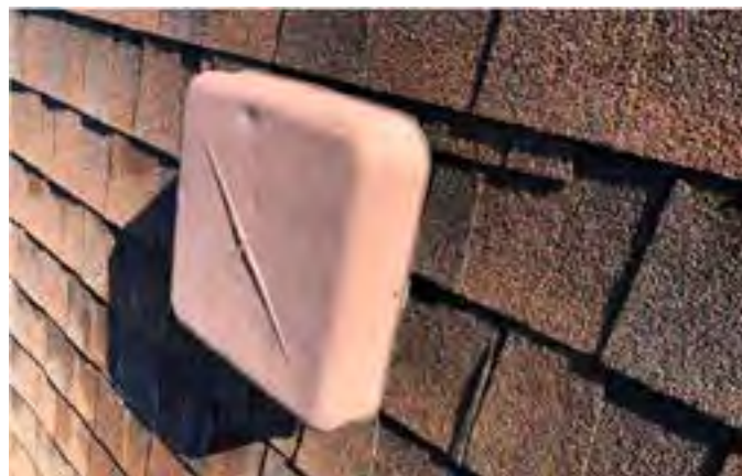
Typical static roof vent near ridge on the Parish Center roof area.
