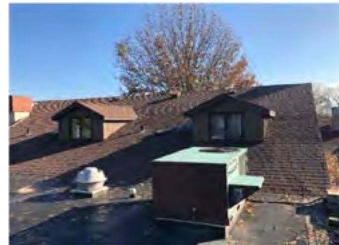
Overview of dormers on west slope of the Parish Center.
