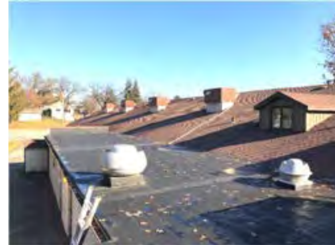
Overview of low-slope EPDM roof system and west slope of the Parish Center.
