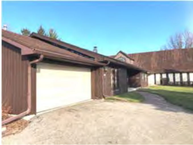
East elevation of Rectory/Parish Offices.
