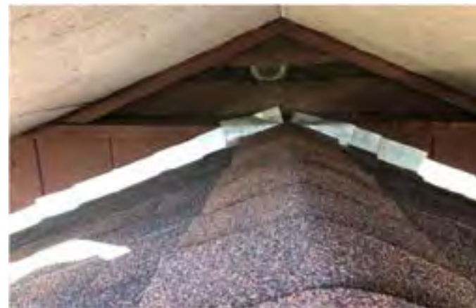
Gable vent at garage rake edge overhang.
