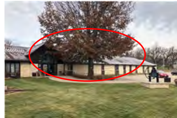
Overview of the east slope on the Parish Center. Some hot spots were observed.
