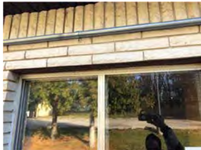
Typical lintel condition at windows. Lintels are in good shape.
