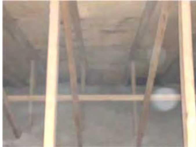
View of east slope of interior attic space, no moisture stains observed.
