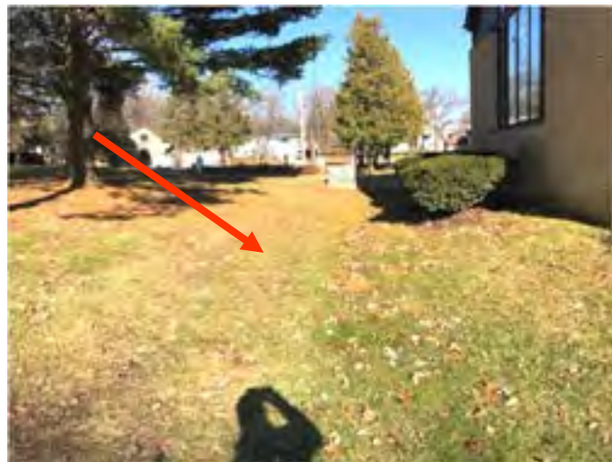
The culvert runs behind the chapel to the back (west side) parking driveway behind the Parish Center.
