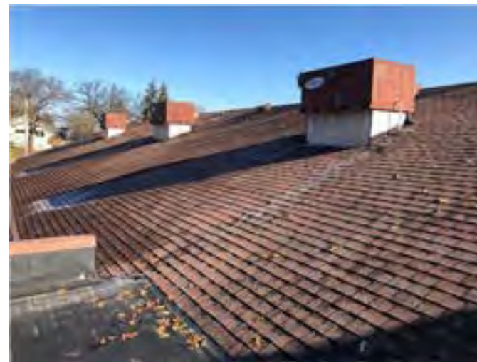
View of west roof slope over the Parish Center.
