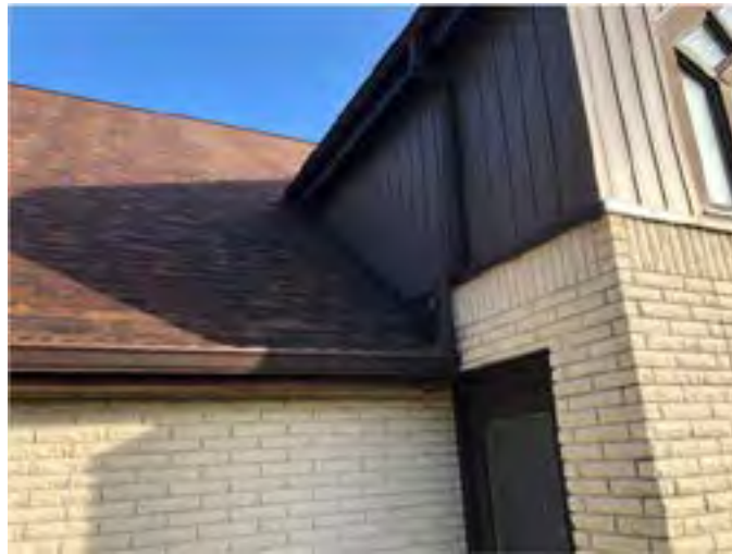
Roof-to-wall transition on south elevation of the Church
