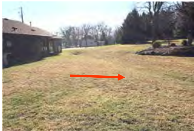
Culvert at rear (west side) of Church.
