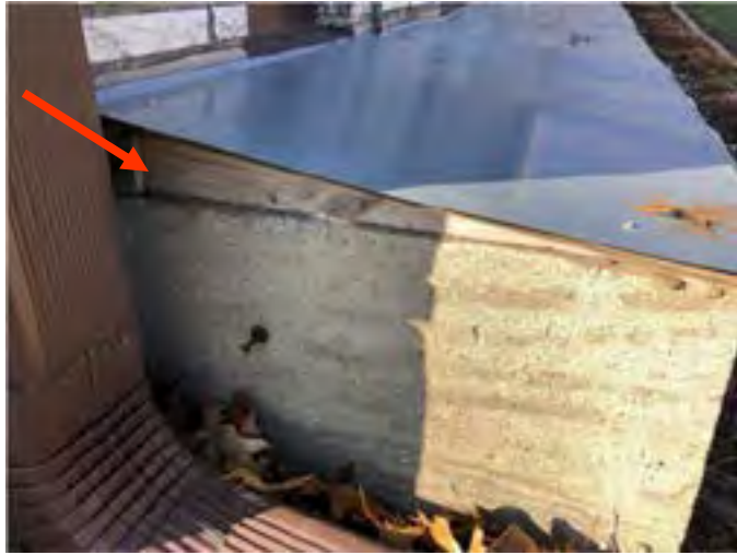
Wood framing observed under sheet metal flashing cover.
