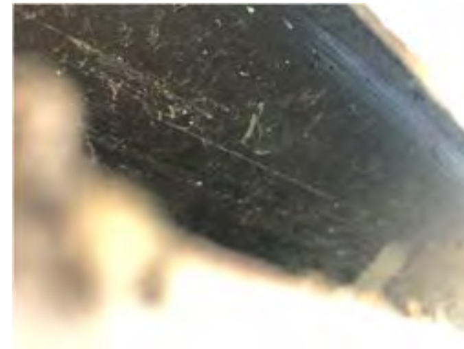
Weather resistive barrier observed behind metal wall panels.
