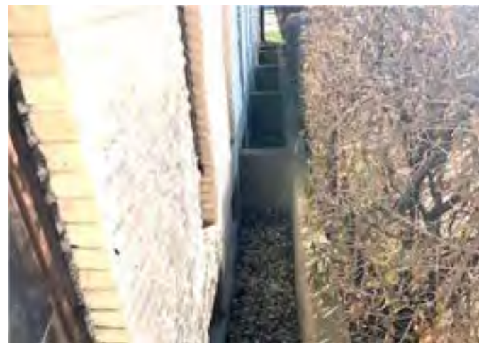
Light well on south side of the Church
