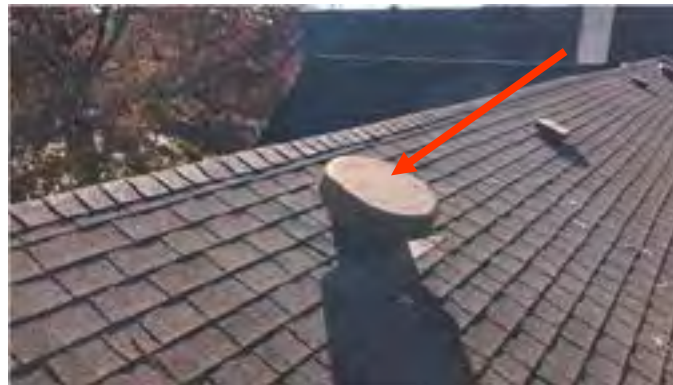
Typical power vent near ridge on the Parish Center roof area.
