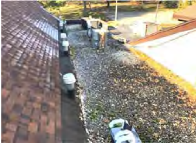
Overview of stone ballasted EPDM roof area facing east.
