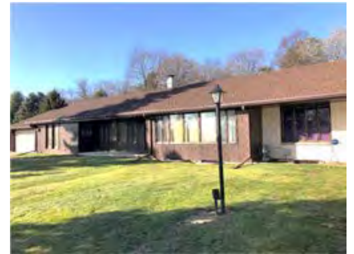
View of east elevation of Rectory/Parish Offices.
