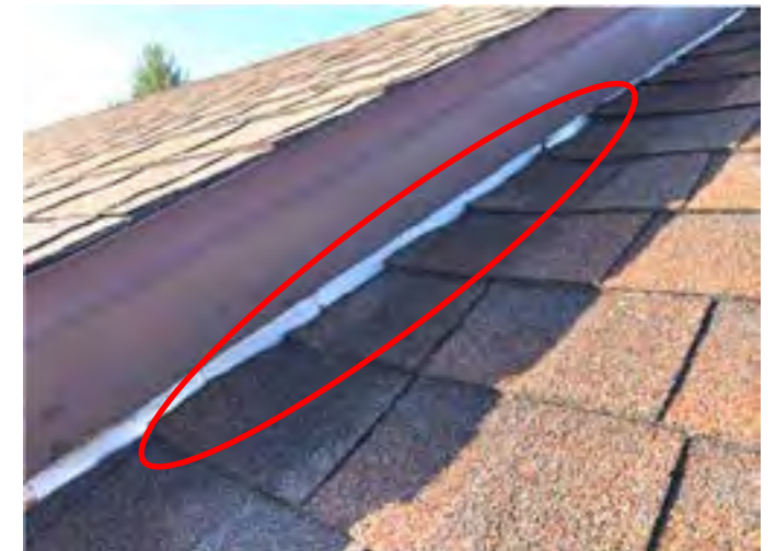
Step flashing observed at change in roof elevation transition at north end of the Parish Center.
