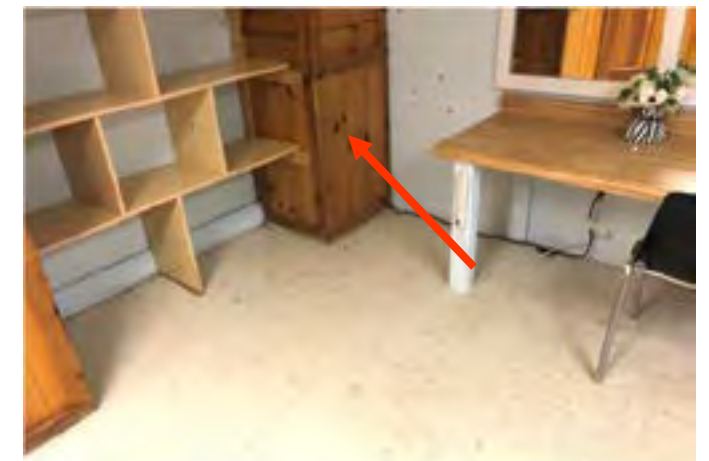
Location of sump pump that appears to be running 24/7. Note: The panel to view the sump pump was inaccessible at the time of our assessment.
