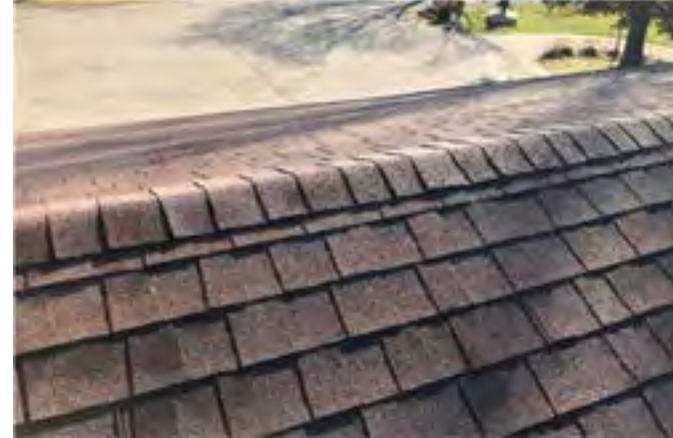
Typical ridge shingle condition on the Parish Center roof area. No ridge vent installed.
