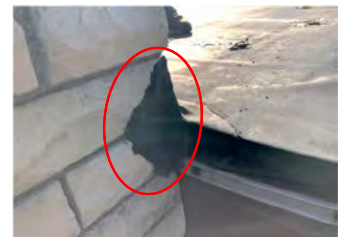
Low-slope roof edge termination is adhered directly to stone masonry
