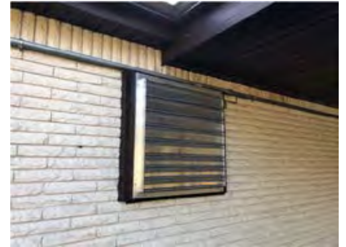
Louver penetration through exterior wall.
