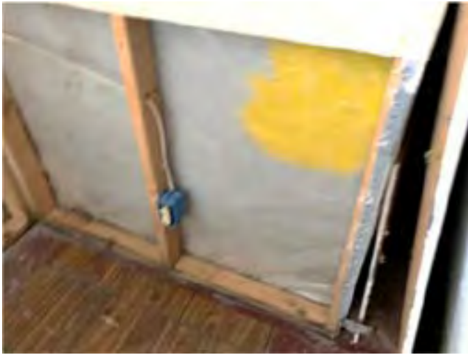
Vapor barrier observed on several interior walls in the basement living quarters.
