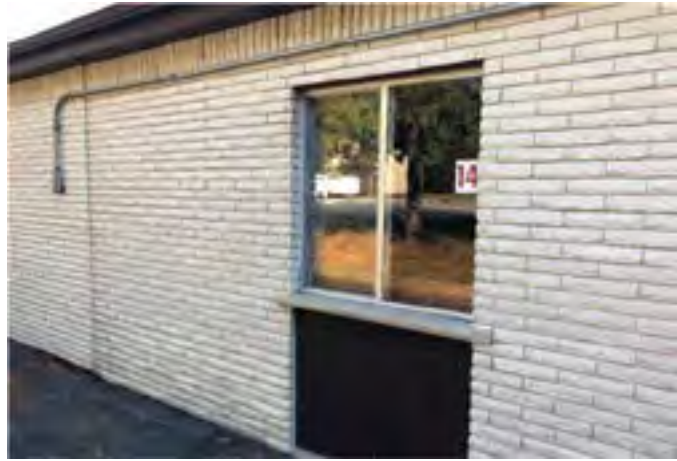
Typical window condition at the Parish Center
