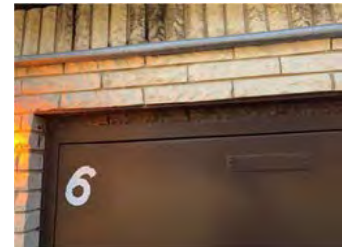
Typical lintel condition at exterior doors. Lintels are in good shape.
