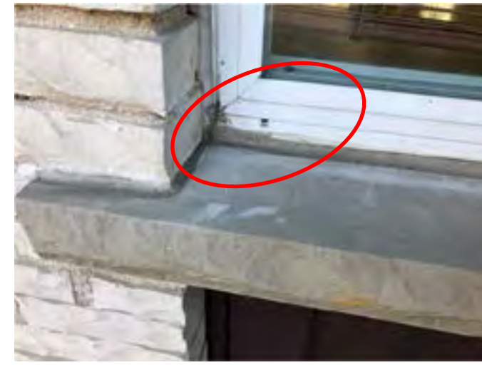
Typical stone window sill condition. Window weeps observed clear of debris.
