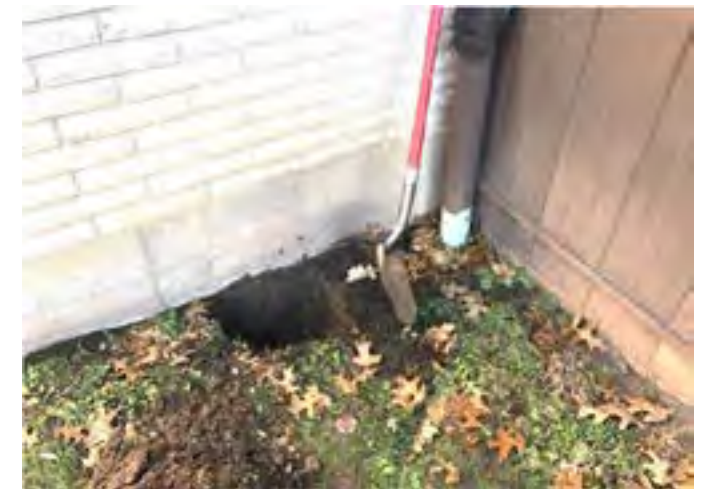
Observation next to foundation of the Church.
