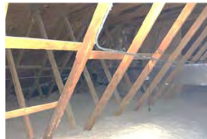
Overview of interior attic space facing northwest.
