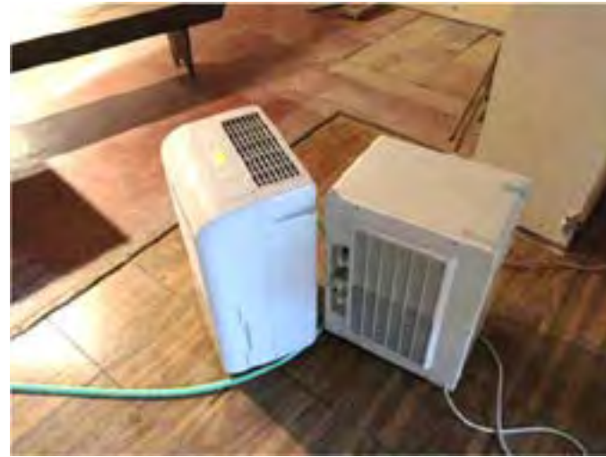
Two dehumidifiers were running at the time of our assessment.
