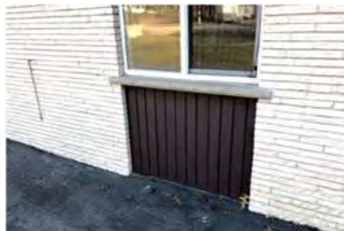
Typical metal panel siding condition at window openings.
