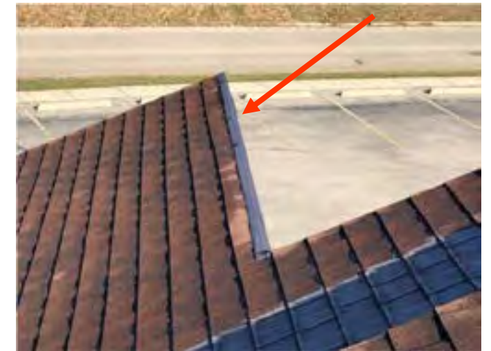
Gutter apron installed at peak of roof at the far north end of the Parish Center.
