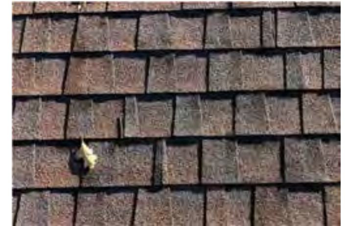
Typical field shingle condition.
