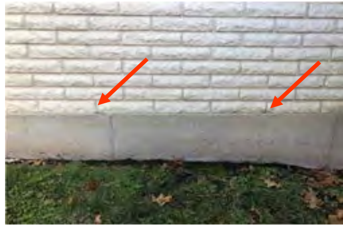
Typical base of wall condition. Weep holes observed.
