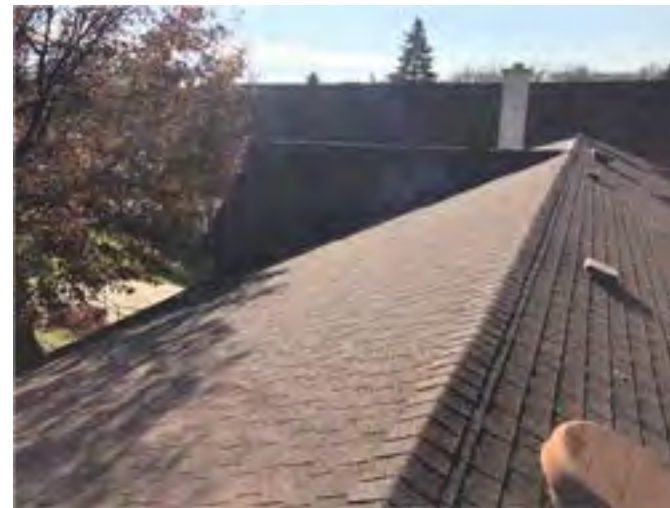
View of east slope of the Parish Center near the Narthex.
