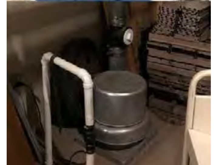
Capped Roof Curb & Removed Roof Exhauster
