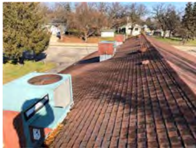
Overview of west roof slope facing north
