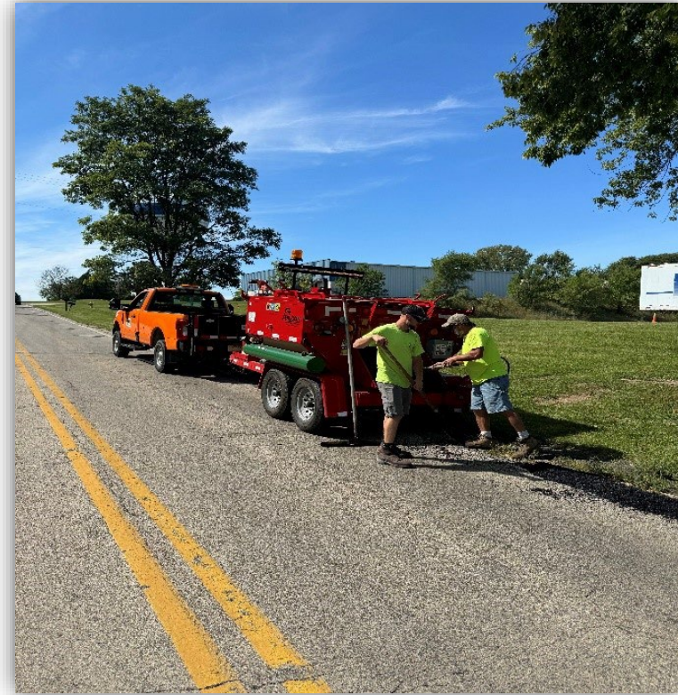
MEMBERS OF THE DEPARTMENT OF PUBLIC WORKS WORK ON CRACK FILLING.
