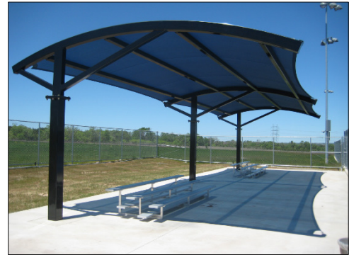
Cantilevered shade structure example
