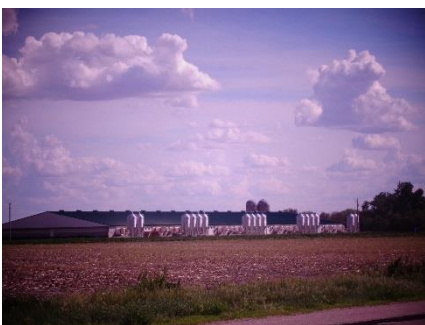
Example of an Animal Confinement Building
