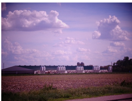
Example of an Animal Confinement Building
