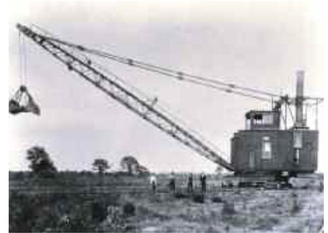
**Figure 3.** First Link-Belt Co. steam powered, wide-gauge, coal handling clamshell crane. Circa 1894. From cover of "Continuous Innovation... For Over 118 Years," Link Belt Construction Equipment Co. Brochure, September 1991.
