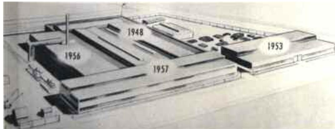
The almost uninterrupted expansion during the past decade of the manufacturing facilities of Link-Belt Speeder Corporation of Cedar Rapids, Iowa, subsidiary of Link-Belt Company is shown in the above architect's drawing. The section marked "1948" doubled the size of the original plant acquired in 1929. The additions in 1953 and 1956 are climaxed by the current expansion which can increase by 40 per cent the company's production of power shovels and cranes.
