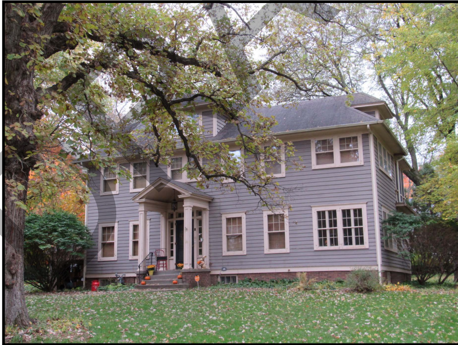
Figure 60. 2237 Washington Avenue SE (57-11443), view to the southwest.
