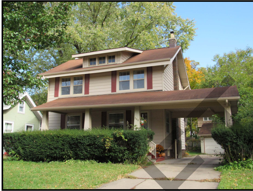
Figure 15. 360 21st Street SE (57-11398), view to the east.
