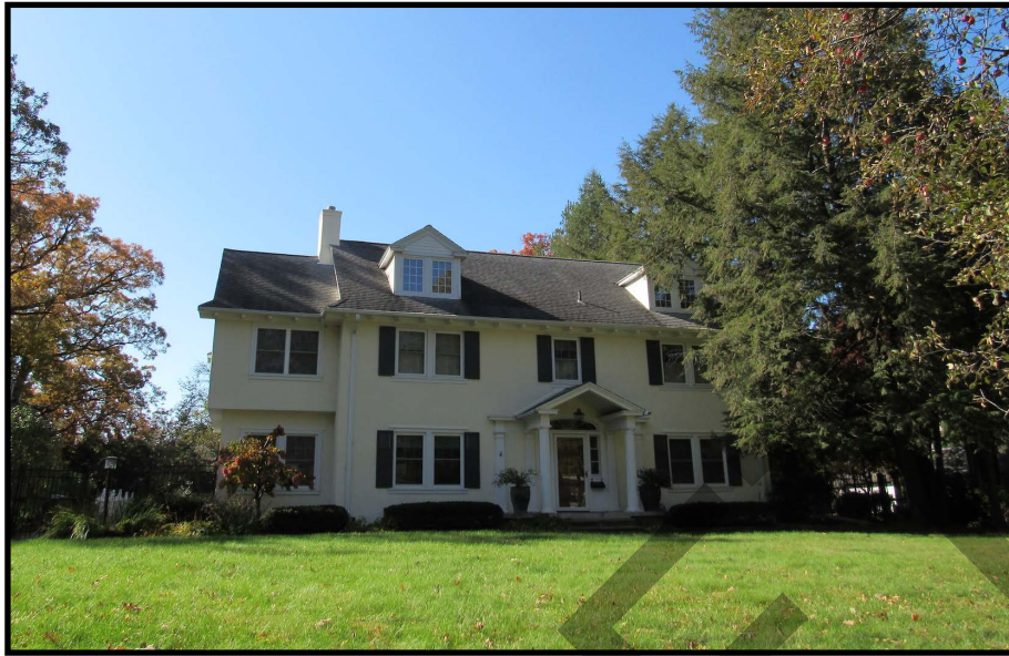
Figure 80. 361 Woodland Drive (57-11463), view to the southwest.
