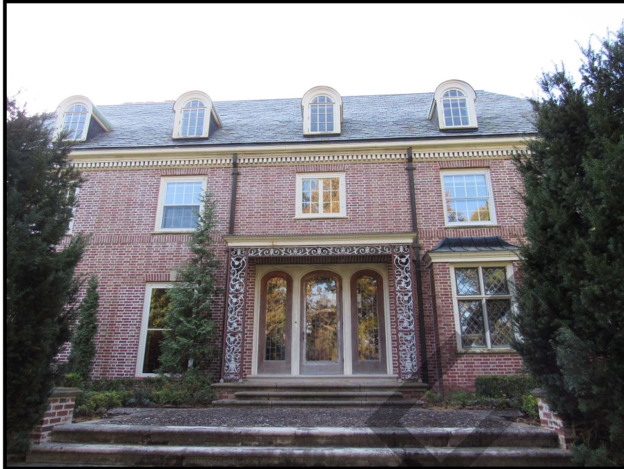
Figure 11. 2101 Grande Avenue SE (57-04013), view to the south.
