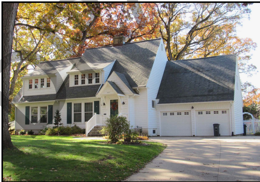
Figure 79. 367 Woodland Drive SE (57-11462), view to the southwest.
