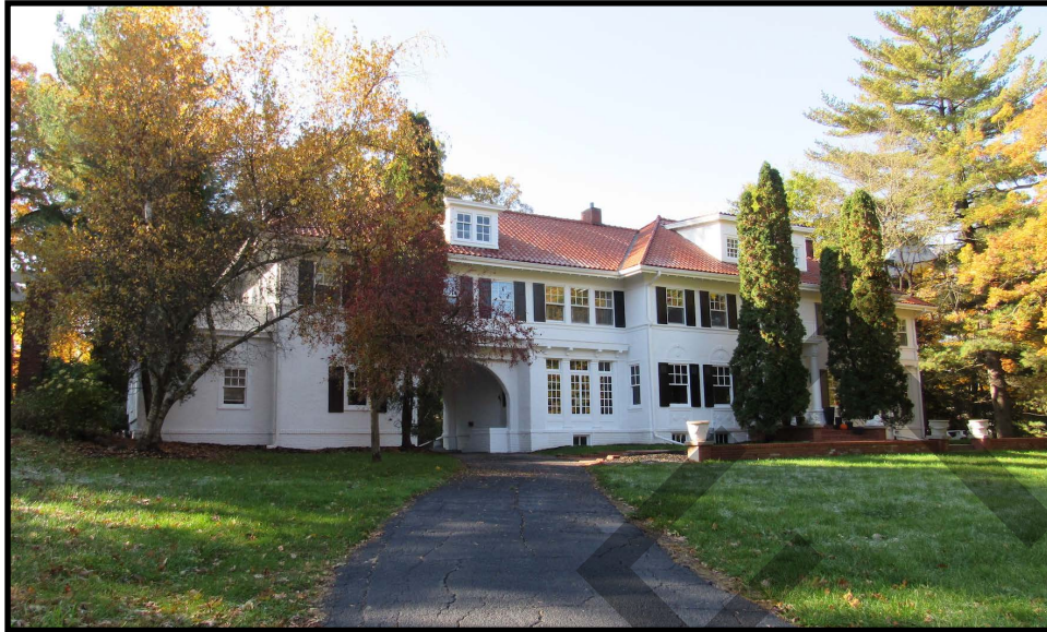
Figure 96. 2317 Grande Avenue SE (57-11479), view to the southwest.
