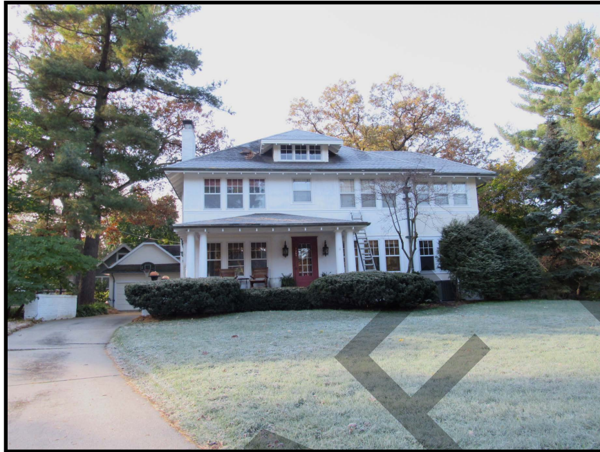
Figure 33. 2207 Grande Avenue SE (57-11416), view to the south.
