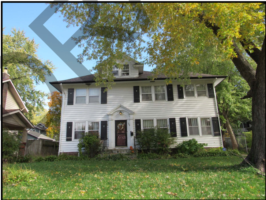
Figure 16. 362 21st Street SE (57-11399), view to the east.
