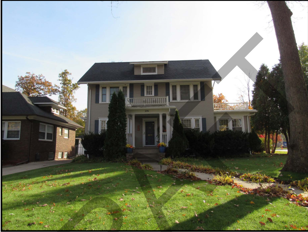
Figure 138. 376 Park Terrace SE (57-11521), view to the east.
