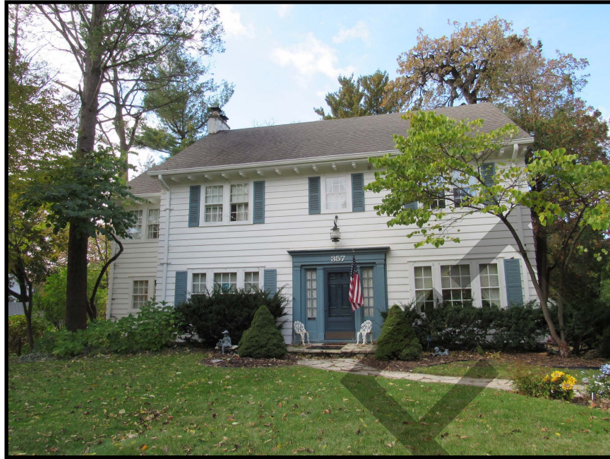
Figure 53. 357 Forest Drive SE (57-11436), view to the west.
