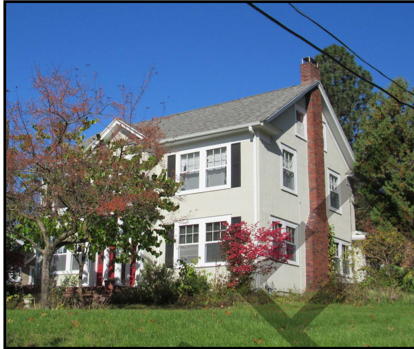
Figure 90. 2424 Bever Avenue SE (57-11473), view to the northwest.
