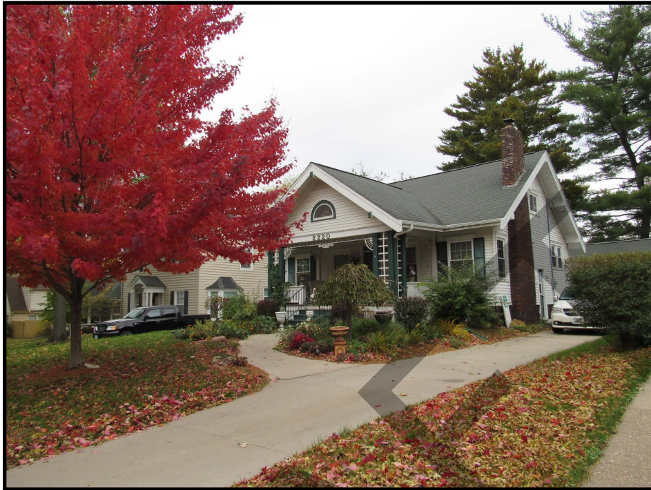
Figure 67. 2220 Bever Avenue SE (57-11450), view to the northwest.
