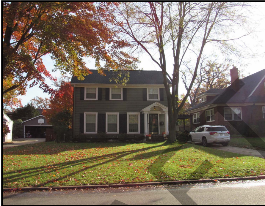
Figure 136. 370 Park Terrace SE (57-11519), view to the east.
