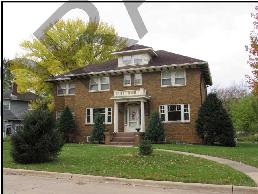
Figure 26. 2101 Washington Avenue SE (57-11409), view to the southwest.
