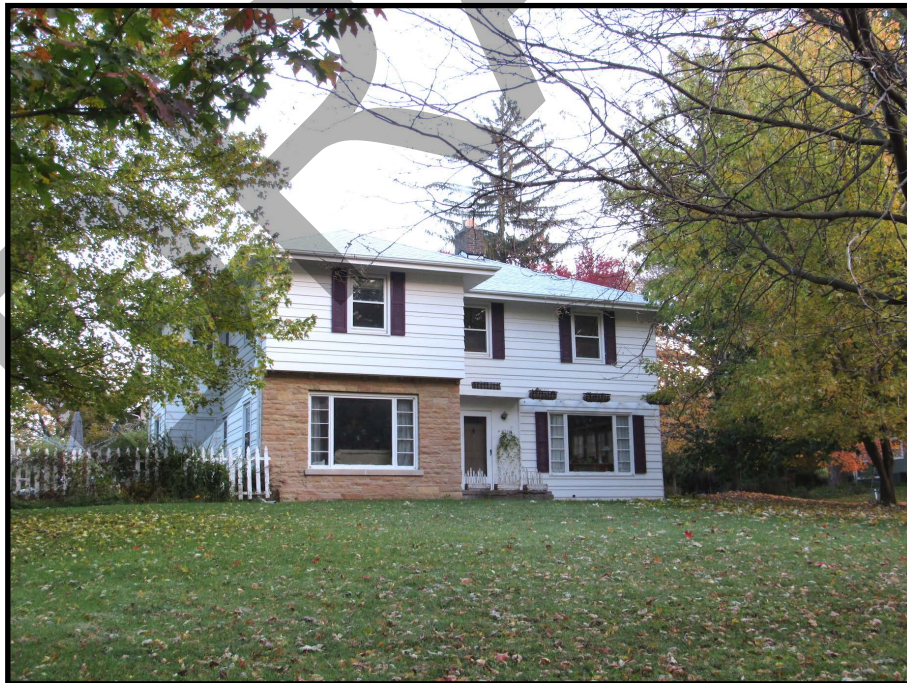
Figure 40. 2220 Washington Avenue SE (57-11423), view to the northeast.
