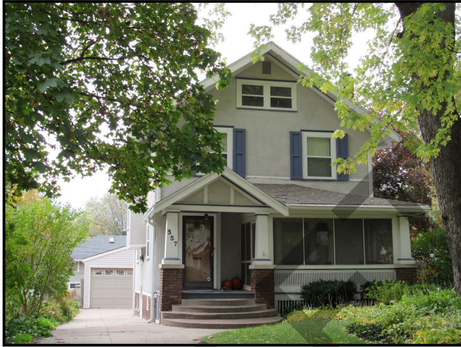
Figure 21. 357 Garden Drive SE (57-11404), view to the west.
