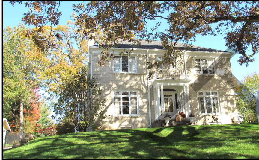
Figure 92. 2434 Bever Avenue SE (57-11475), view to north.
