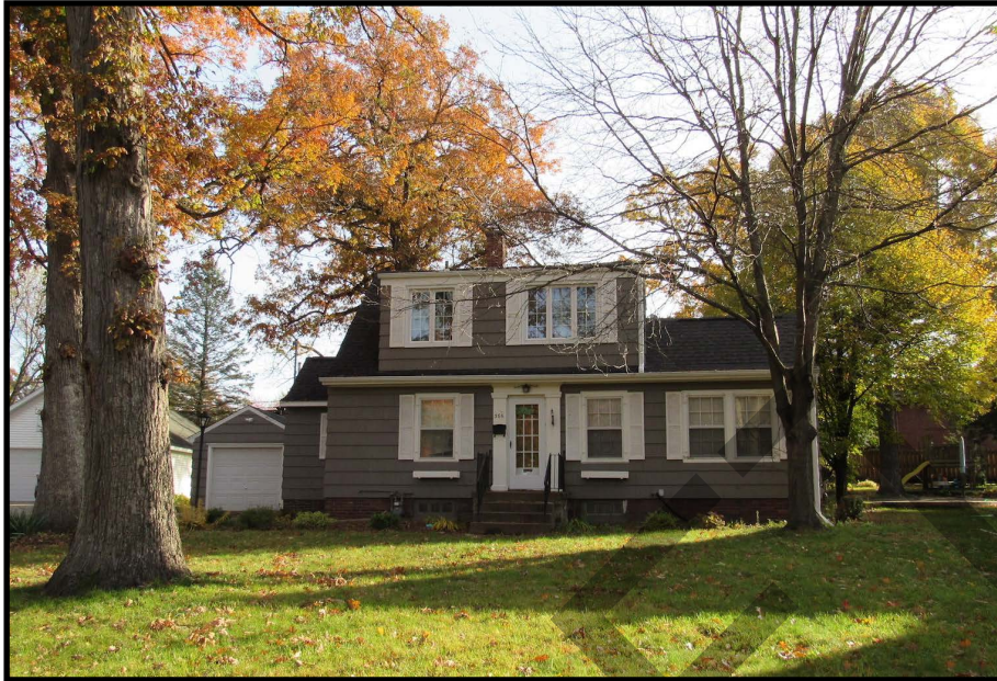
Figure 134. 366 Park Terrace SE (57-11517), view to the east.
