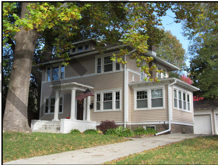
Figure 12. 352 21st Street SE (57-11395), view to the east.
