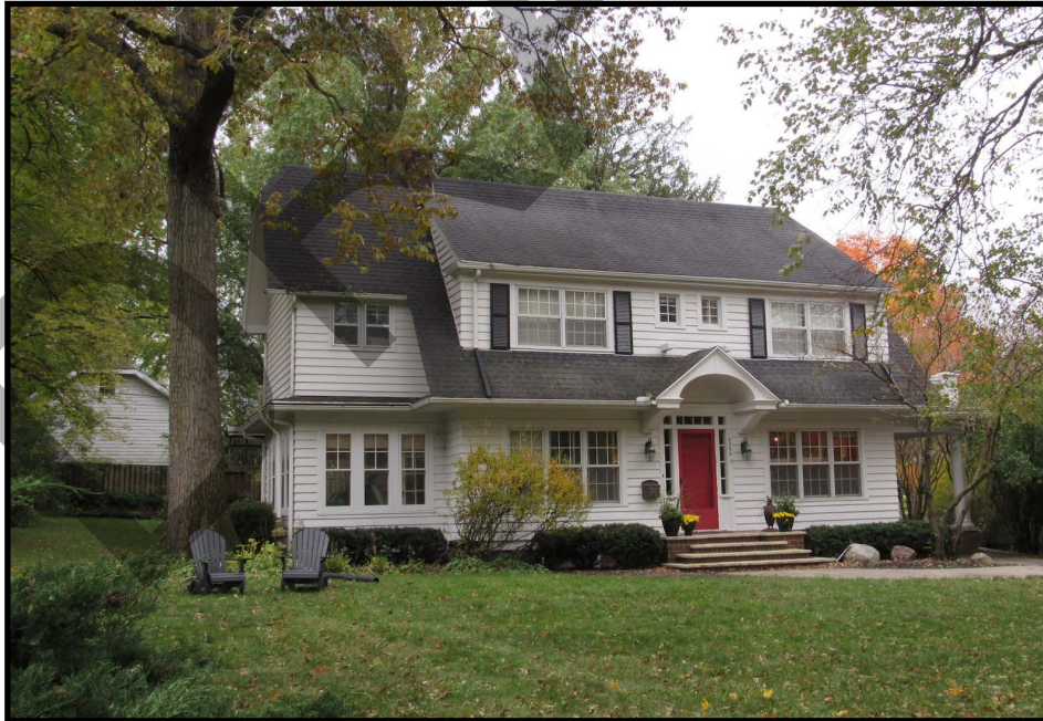
Figure 58. 2259 Washington Avenue SE (57-11441), view to the southwest.
