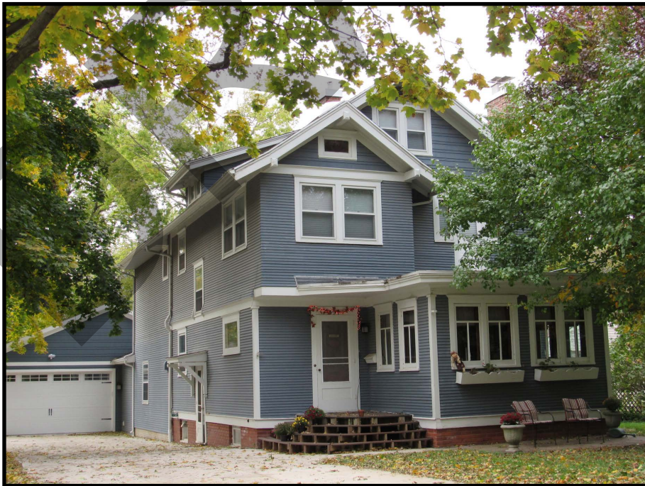
Figure 20. 359 Garden Drive SE (57-11403), view to the northwest.
