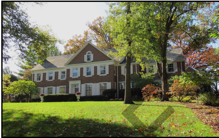
Figure 82. 349 Woodland Drive SE (57-11465), view to southwest.
