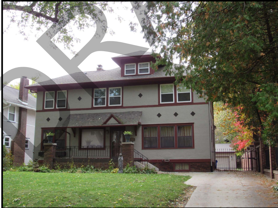
Figure 22. 355 Garden Drive SE (57-11405), view to the west.
