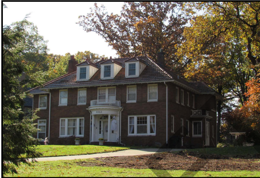
Figure 84. 2343 Grande Avenue SE (57-11467), view to the south.
