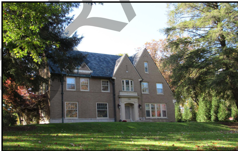
Figure 83. 345 Woodland Drive SE (57-11466), view to the southwest.
