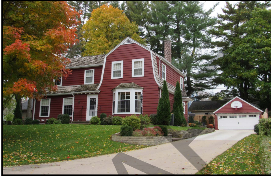
Figure 61. 2227 Washington Avenue SE (57-11444), view to the south.
