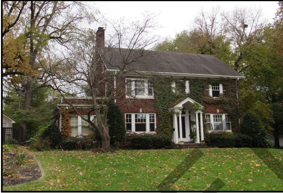
Figure 57. 2267 Washington Avenue SE (57-11440), view to the south.
