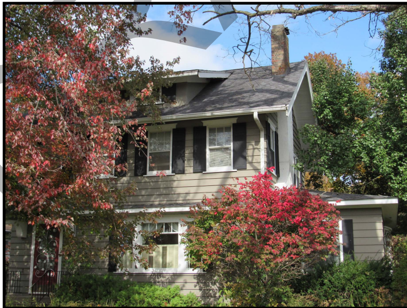
Figure 121. 2618 Bever Avenue SE (57-11504), view to the northwest.
