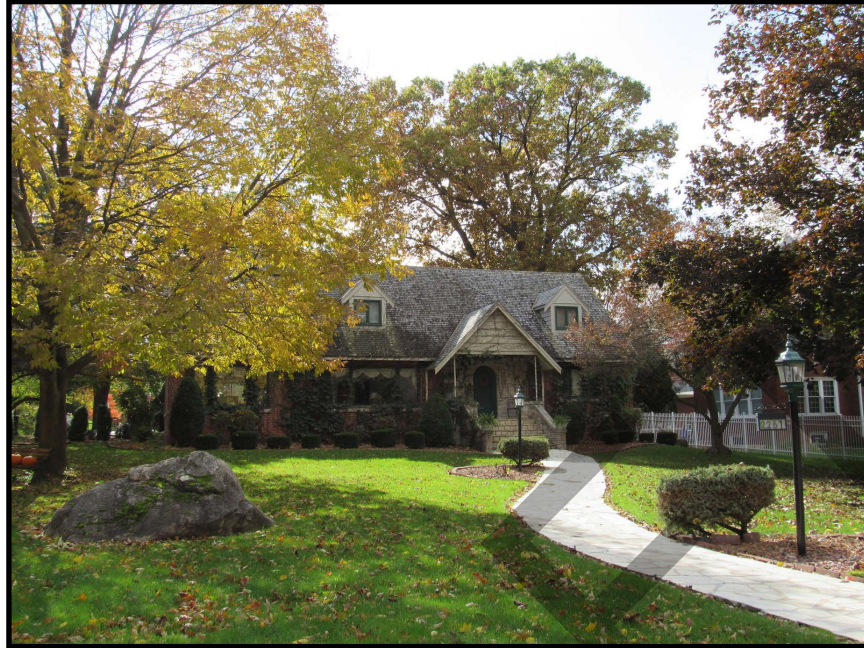
Figure 45. 2261 Grande Avenue SE (57-11428), view to the southwest.
