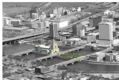
Aerial view of building site
