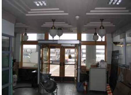
North tower lobby: before
