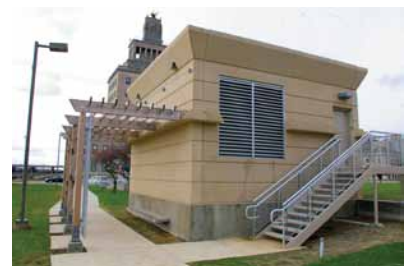
New generator building
