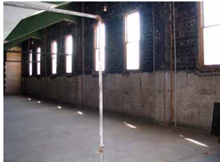
Conference rooms (mezzanine level): before
