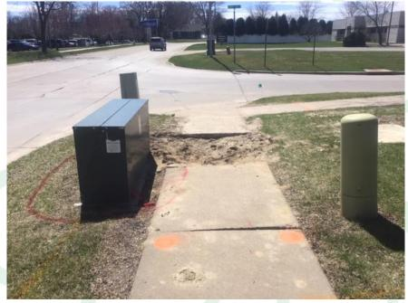
Debris left after job completion • Emergency utility repair. No permit, no area protection.
