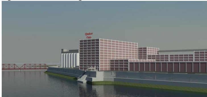
Figure III - 2: Rendering of floodwall at Quaker Oats Plant
