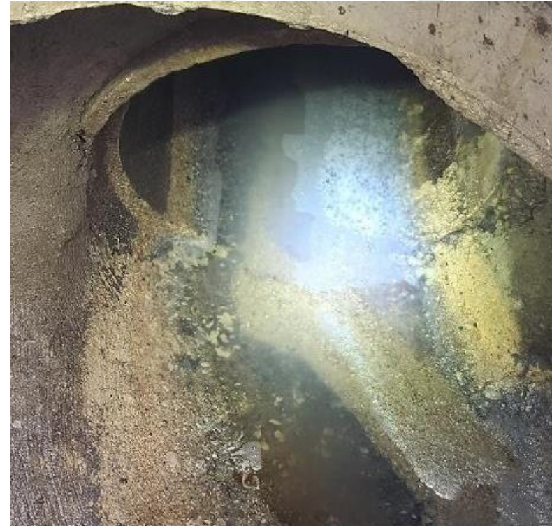
Soap bubbles led to the discovery of laundry facility discharge from Coe College
