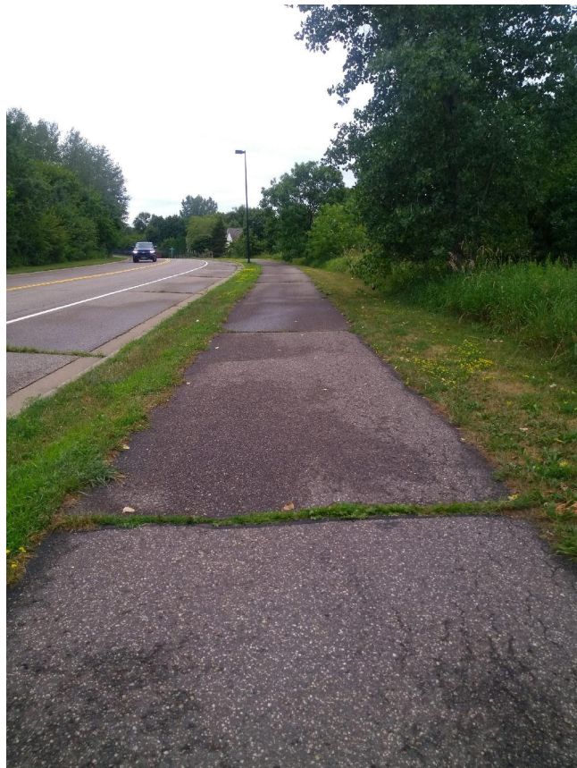
FIGURE 3.38 An example of a trail that would benefit from crack and surface treatments.
