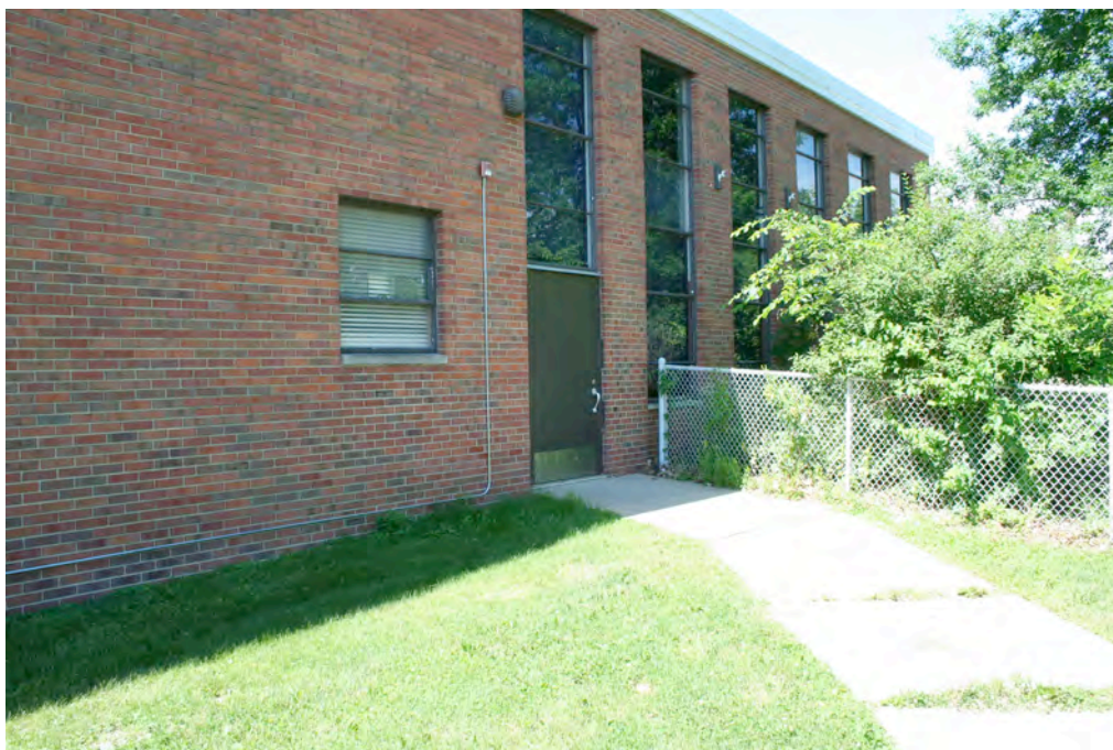
Figure 11. (Image 0013) Monroe Elementary, Section A, North Elevation – 2014
