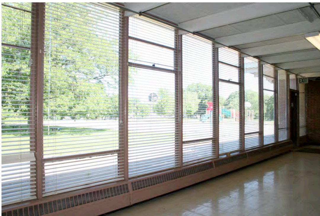
Figure 13. (Image 0018) Monroe Elementary, Typical Windows – 2014
