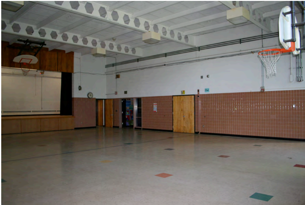
Figure 16. (Image 0023) Monroe Elementary, Section A, Multi-Purpose Space – 2014
