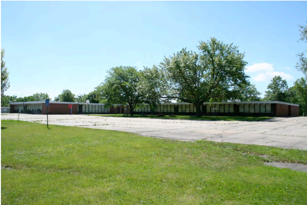
Figure 9. (Image 0010) Monroe Elementary, Rear (North) Elevation – 2014
