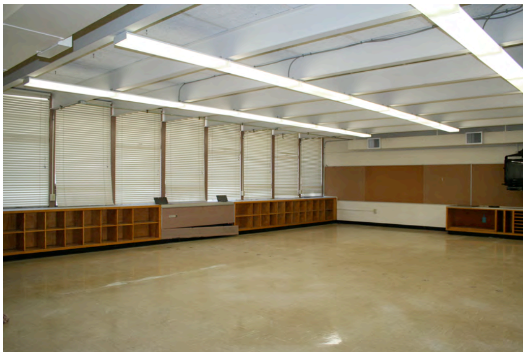
View of the same classroom, looking southeast.
