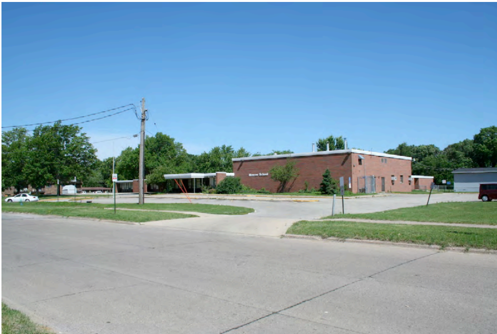
Figure 8. (Image 0007) Monroe Elementary, Primary (South) Elevation - 2014
