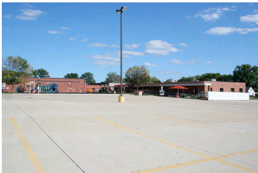
View of the rear elevations.
