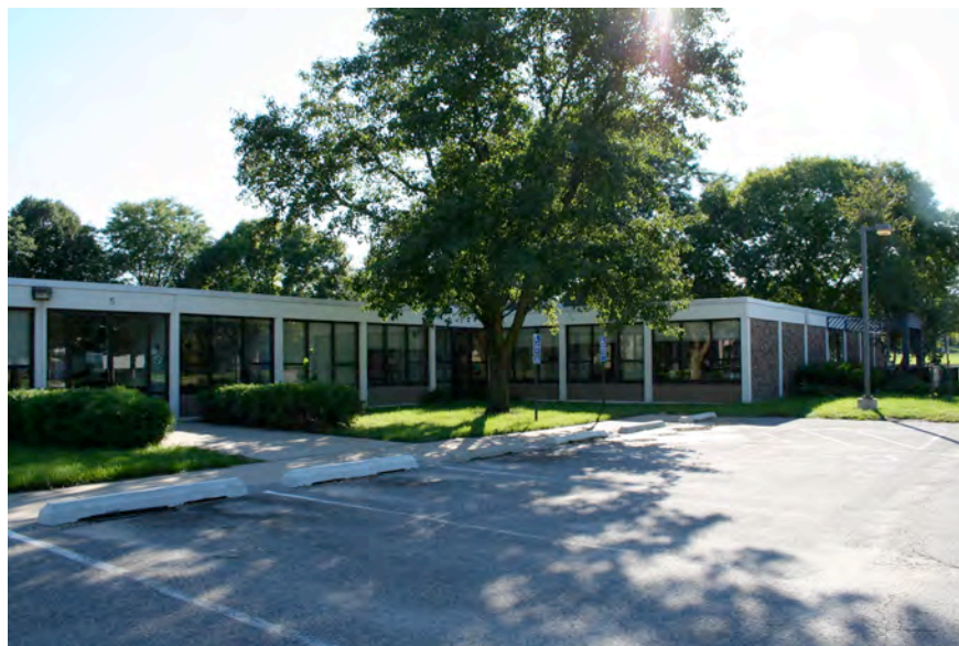
View of the classroom wing.
