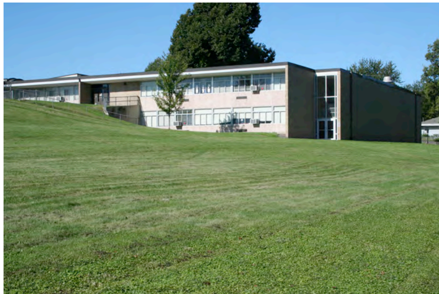
View of the classroom wing.
