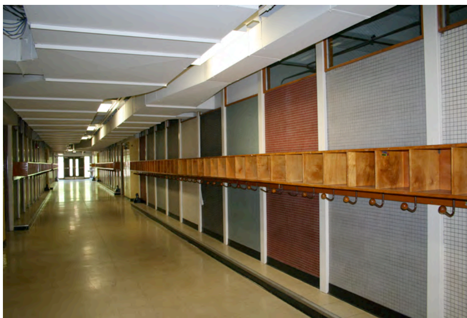
Figure 22. (Image 0019) Monroe Elementary, Typical Hallway – 2014
